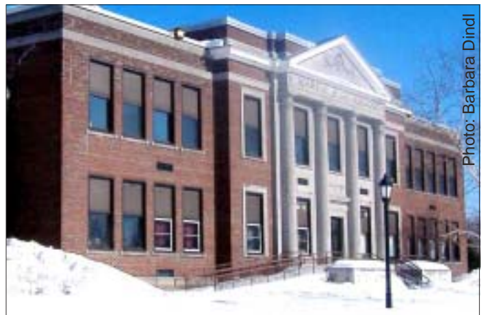
A school outside of Fort Drum was renovated and turned into affordable housing for military families.
