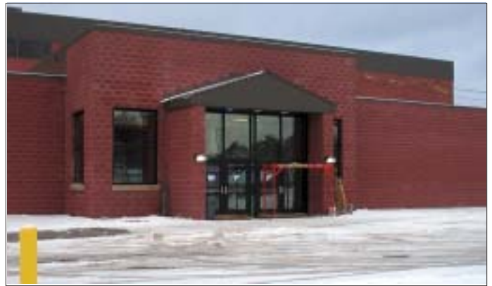
The new Pine Plains Physical Fitness Center, Fort Drum, N.Y.
