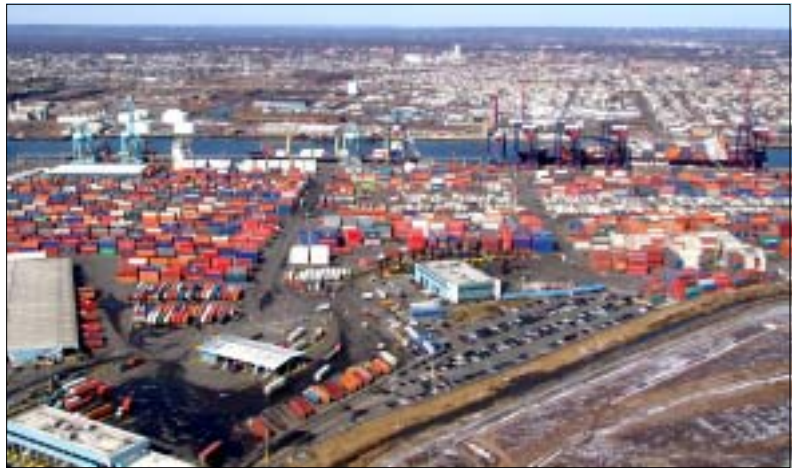
New York Container Terminal, formerly known as Howland Hook Terminal on Staten Island, N.Y. In keeping with its mission to create a world-class harbor, the Corps and the Port Authority, along with other sponsors, are deepening the channels to ensure that the harbor is able to safely and efficiently accommodate the new megaships that are entering the port.
