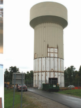
Water Tower Raising
