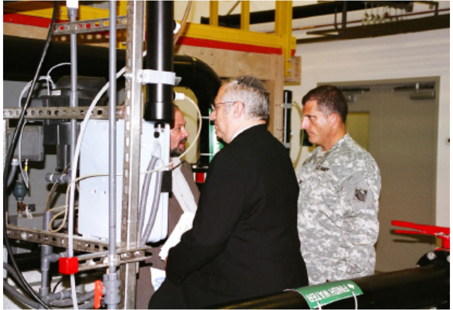
Prior to the ribbon cutting ceremony, Col. Nello Tortora and Alan Steinberg tour the inside of the plant and observe the water treatment operations.
