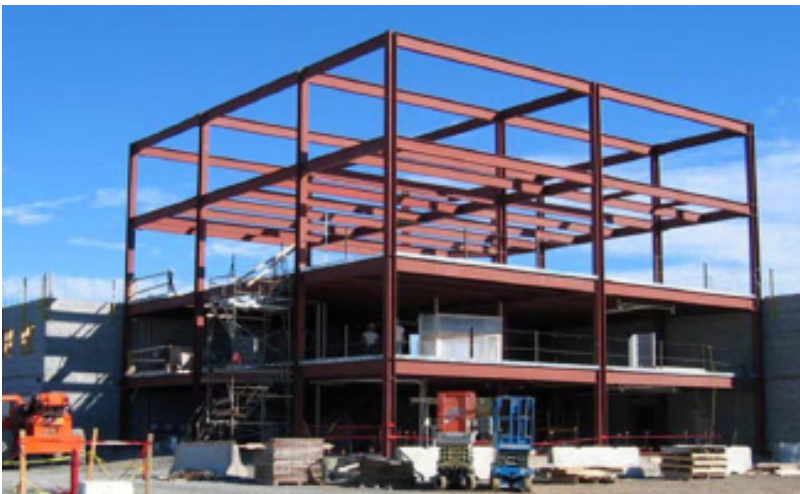
The 10100 Barracks project during construction at Fort Drum, NY.
