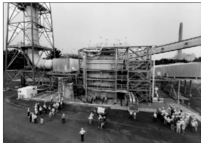
▲ The unique Jet Bubbling Reactor® (center) was constructed from fiberglass-reinforced plastic.
