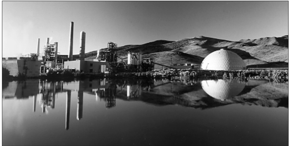
▲ SPPC's Piñon Pine project demonstrates air-blown, fluidized-bed IGCC technology using hot gas cleanup, and evaluates a low-Btu gas combustion turbine.
