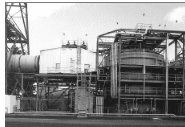
▲ Unique CT-121 SO 2 scrubber at Plant Yates combined a number of functions and eliminated process steps.
