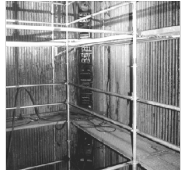
▲ A portion of ABB Combustion Engineering's Low-NO x Concentric Firing System (LNCFS™) is shown being installed on a tangentially-fired boiler.
