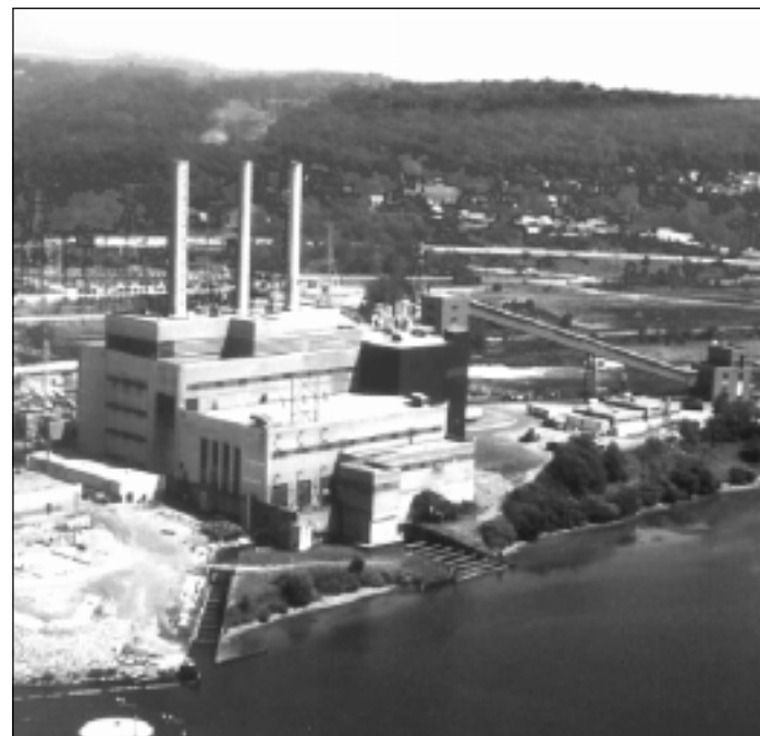
▲ The PFBC demonstration at the repowered 70-MWe unit at Ohio Power's Tidd Plant led to significant refinements and understanding of the technology.
