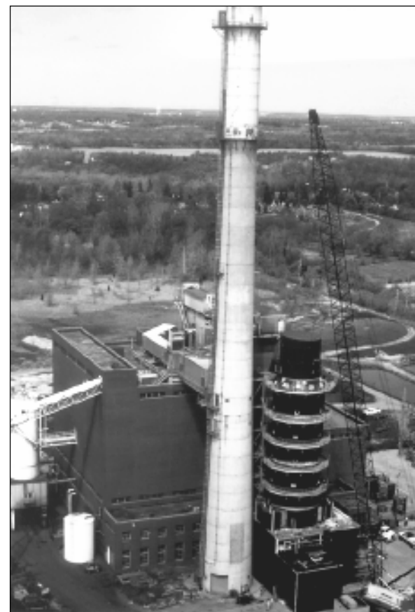
▲ The LIFAC system successfully demonstrated at Whitewater Valley Station Unit No. 2 is being retained by Richmond Power & Light for commercial use with high-sulfur coal. There are 10 full-scale LIFAC units in Canada, China, Finland, Russia, and the United States.
