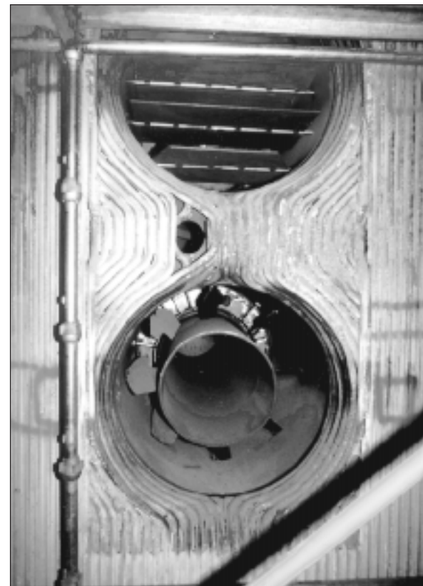
▲ The LNCB® is viewed from within the boiler.
