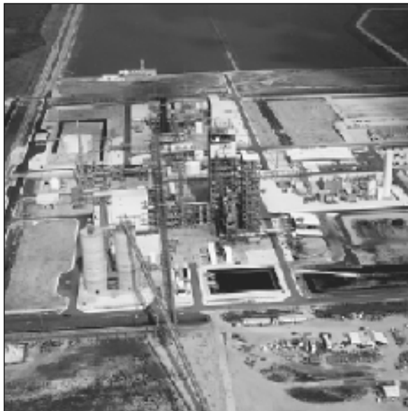
▲ Tampa Electric Company's Polk Power Station Unit 1, a 250-MWe IGCC greenfield installation, is currently in operation. It is one of the world's cleanest and most advanced coal power plants.
