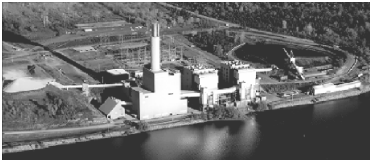
▲ New York State Electric & Gas Corporation's Milliken Station is hosting the demonstration of a combination of unique SO 2 and NO x control technologies.
