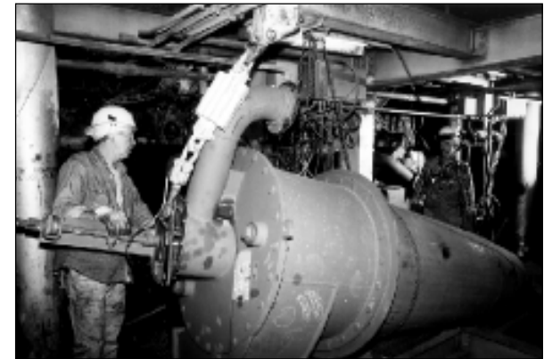
▲ NO x emissions at Georgia Power's Plant Hammond were reduced by 63 percent with Foster Wheeler's low-NO x burners, shown here, and advanced overfire air.
