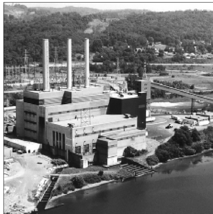
▲ The PFBC demonstration at the repowered 70-MWe unit at Ohio Power's Tidd Plant led to significant refinements and understanding of the technology.
