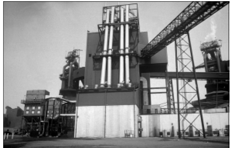
▲ Shown here is the completed Bethlehem Steel Corporation facility to demonstrate the injection of granulated coal directly into two blast furnaces at Burns Harbor, IN.
