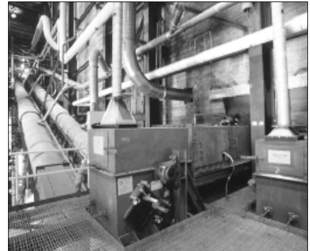
▲ Coal and sorbent conveyors can be seen just after entering the Tidd Plant.
