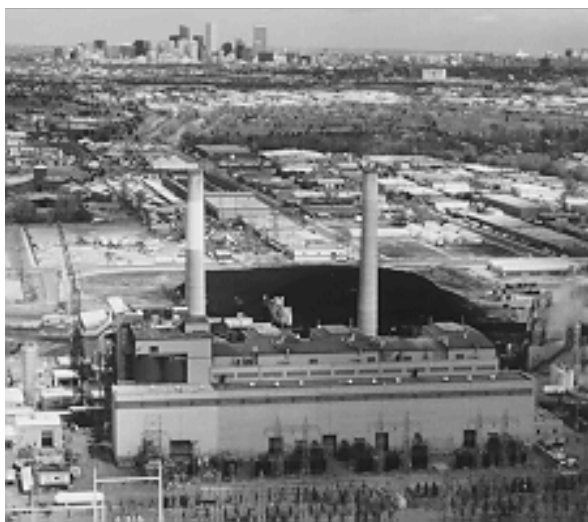
▲ Public Service Company of Colorado demonstrated low-NO x burners, induct injection, and SNCR at Arapahoe Station near Denver.
