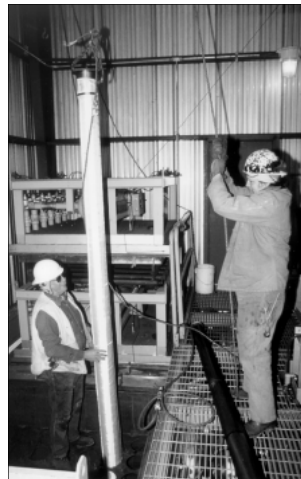
▲ Workers lower one of the catalyst holder tubes into a mounting plate in the penthouse of the high-temperature baghouse.
