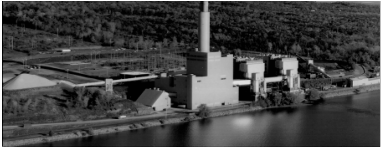
▲ New York State Electric & Gas Corporation's Milliken Station is hosting the demonstration of a combination of unique SO 2 and NO x control technologies.
