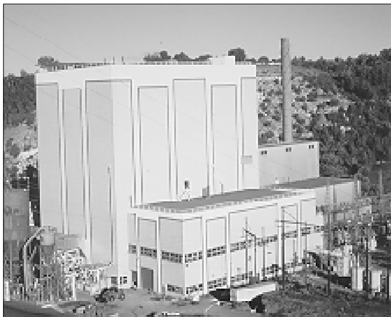
▲ The 110-MWe Nucla ACFB demonstration enabled Pyropower Corporation (now owned by Foster Wheeler) to save almost 3 years in establishing a commercial line of ACFB units.
