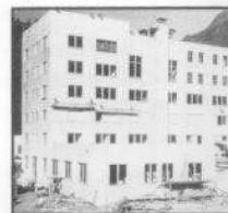
Federal Building, Ketchikan, Alaska.
