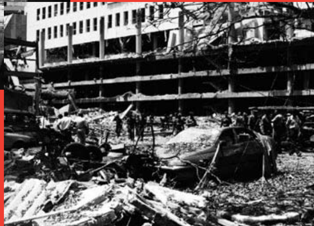
Above: Galadari car park looking from the entrance towards the blast site.
