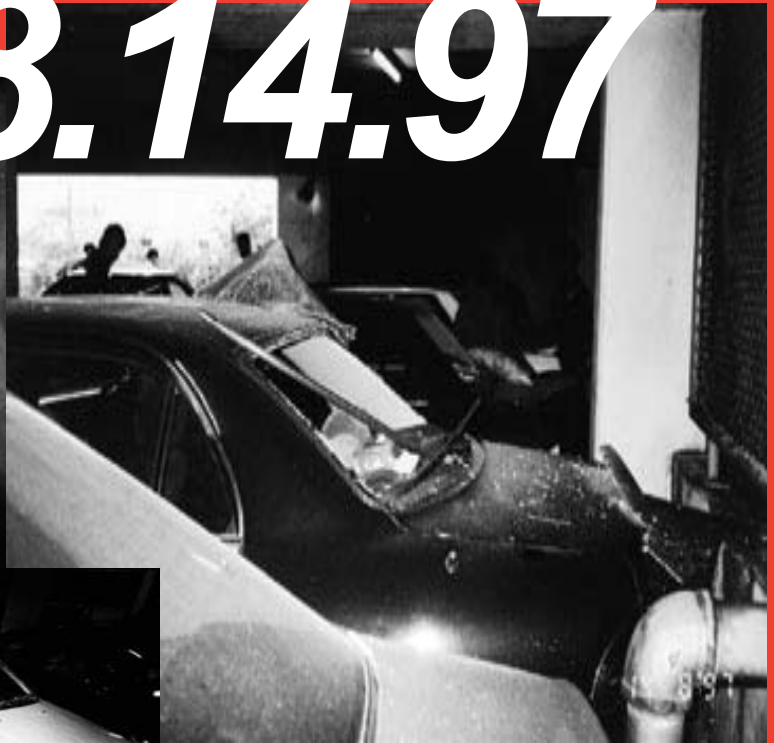
Damage to a car in the parking garage of the IBM building.
