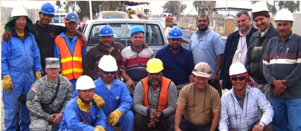
Wayne Birgado right, in brown hard hat) and road construction crew in Baghdad.
