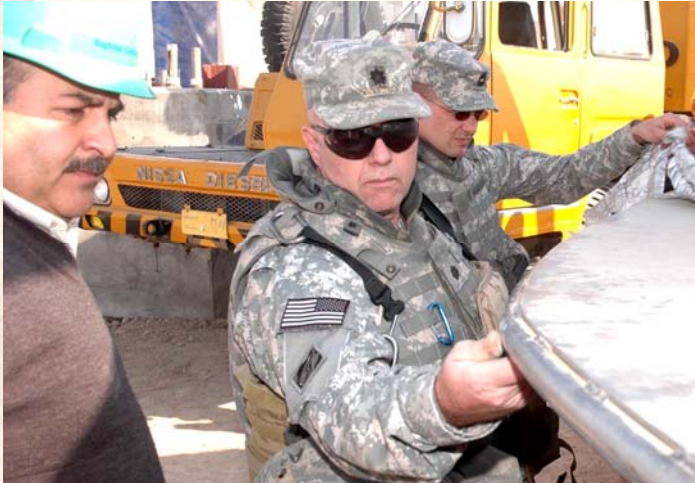
At a $160 million expansion project on the Qudas electric generating facility north of Baghdad, CDR Frost inspects the diffuser.
