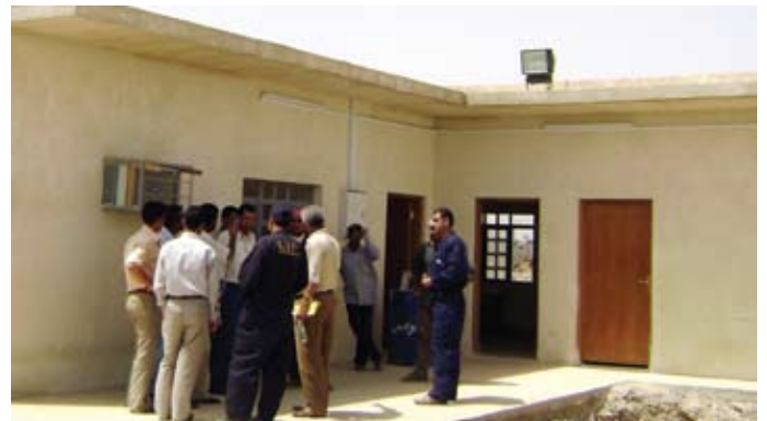
After: Plant management now oversees operations from the rehabilitated facility.
