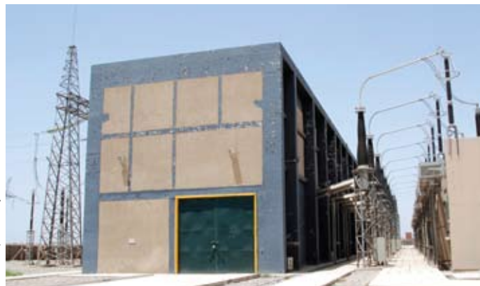
The 400 kV Gas Insulated Switchgear is housed indoors and connects the 400 kV transmission lines from the Baghdad ring with 132 kV distribution lines.
