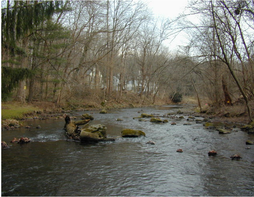
View looking downstream at the reach of Monocacy Creek containing cross section at station 91, February 25, 2002.
