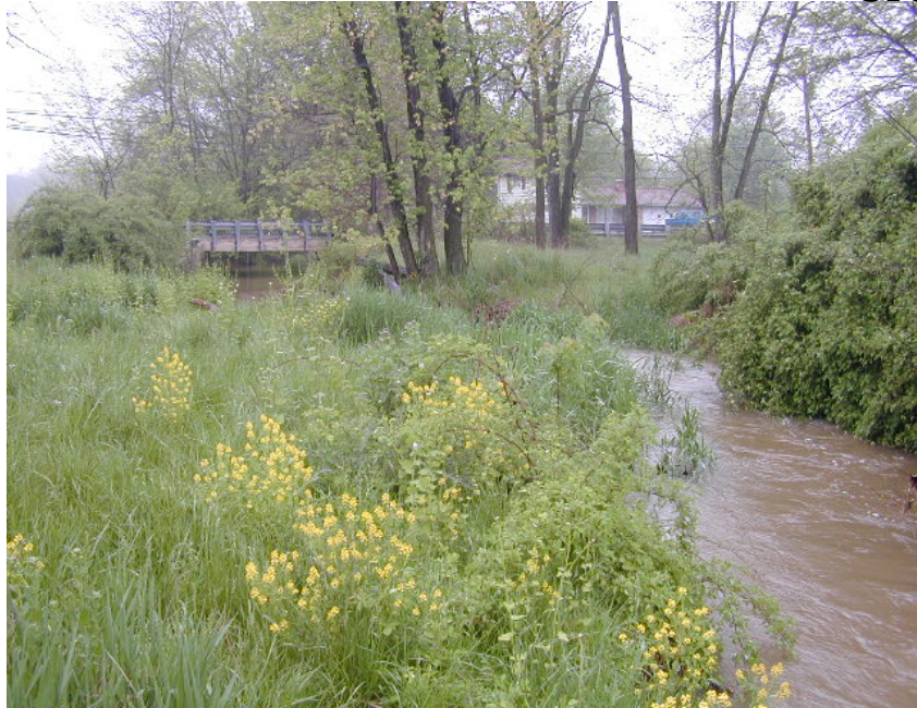
View looking upstream at the reach of Newburg Run containing cross section at station 82, May 9, 2002.
