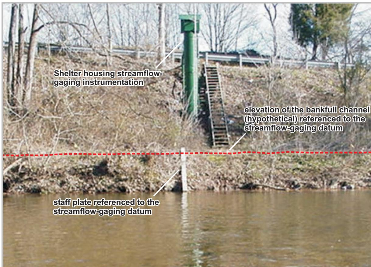
**Figure 2.** Streamflow-gaging station and hypothetical example of a bankfull-channel elevation used for development of regional curves in Pennsylvania and selected areas of Maryland. Photograph taken by Kirk E. White, U.S. Geological Survey, January 2000.
