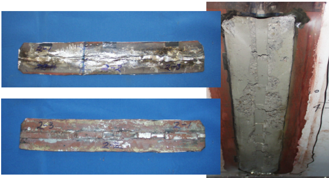
Figure 5.87 Liner Specimen at Tear #2
