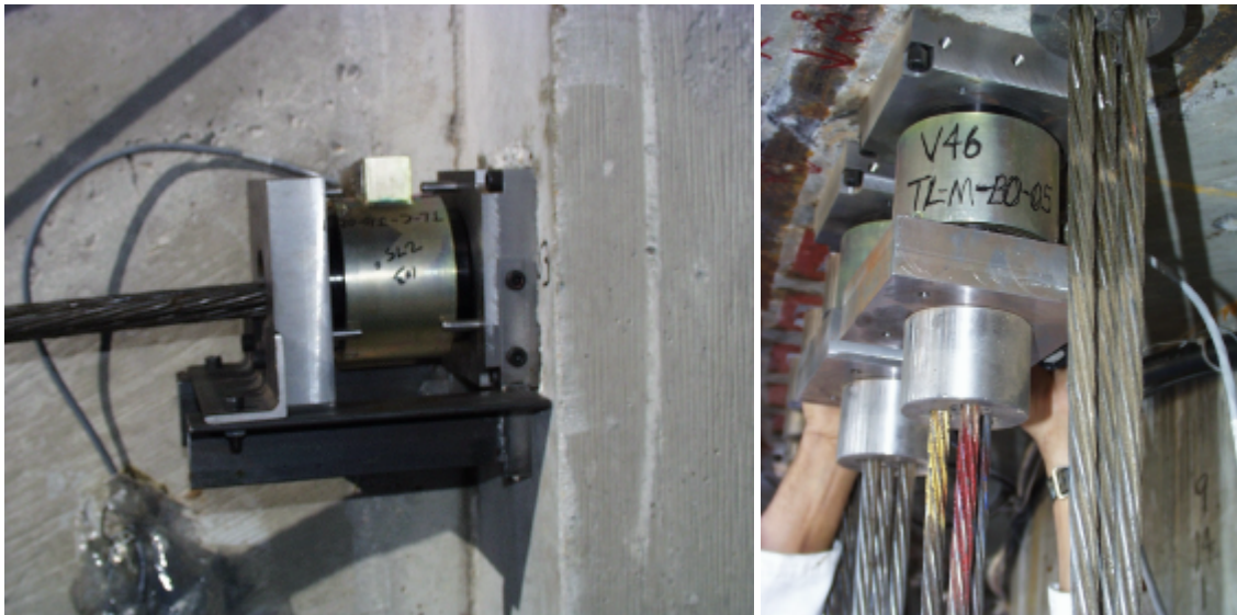
Figure 3.14 Geokon Load Cell (a) Installation Jig, (b) In-Place
