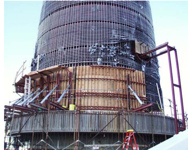
Figure 2.46 C1 Formwork Installation
