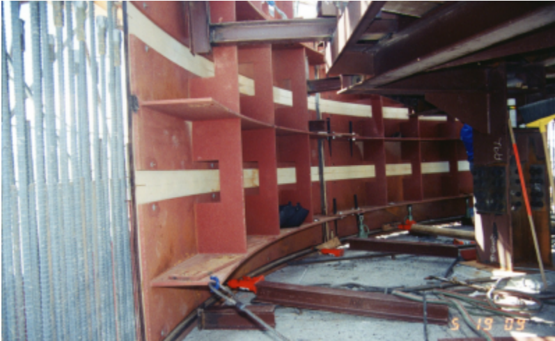
Figure 2.36 Liner Panels with Jigs
