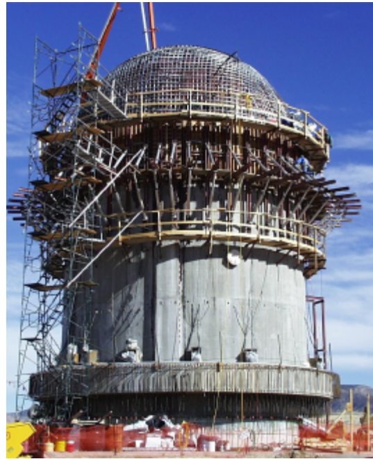
Figure 2.50 C4 Concrete Placement
