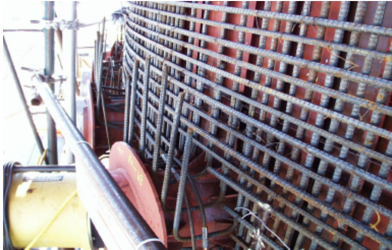
Figure 2.40 Inner Rebar at M/S Penetrations
