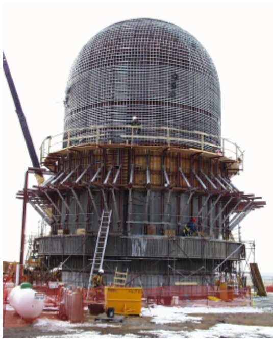
Figure 2.49 C2 Formwork
