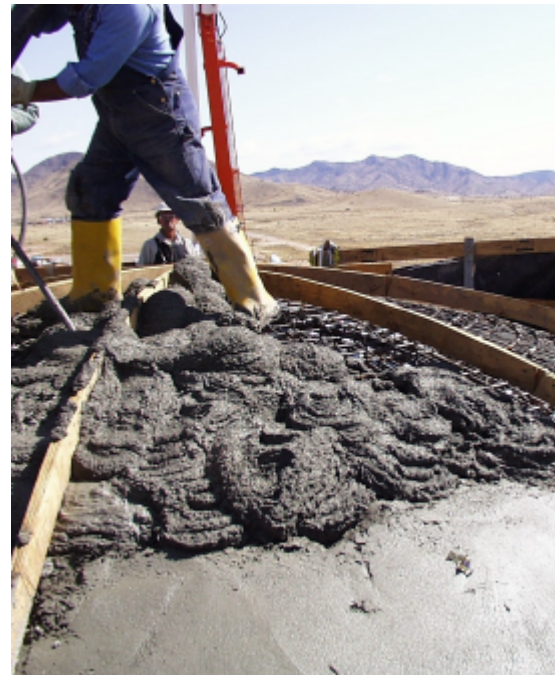
Figure 2.52 D3 Concrete Placement
