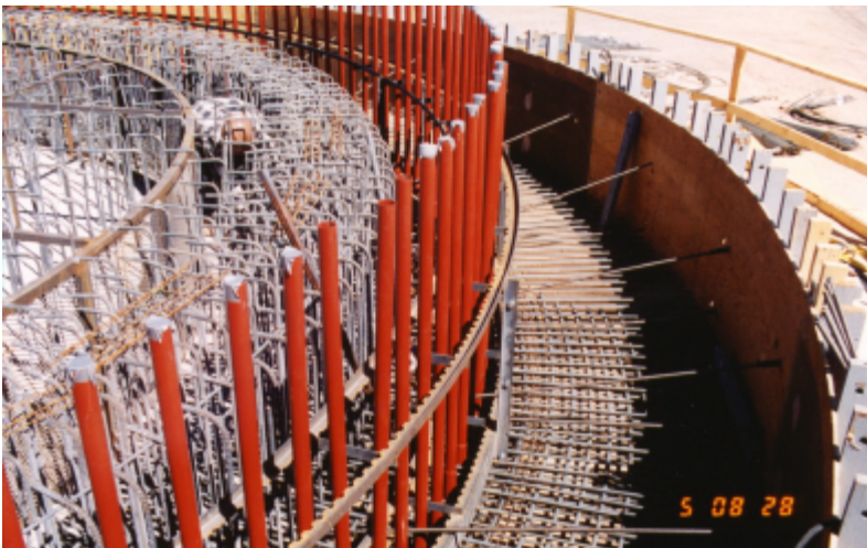
Figure 2.22 F3 Rebar and Formwork
