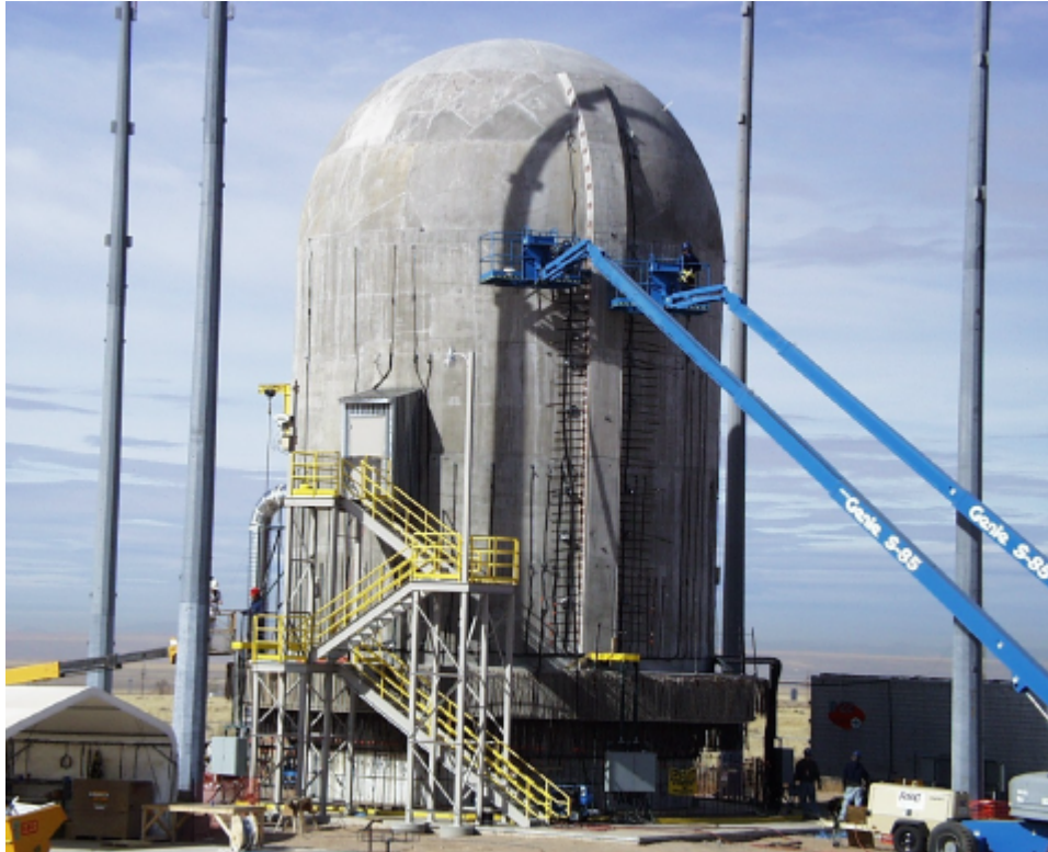
Figure 2.57 Tensioning Hoop Tendons
