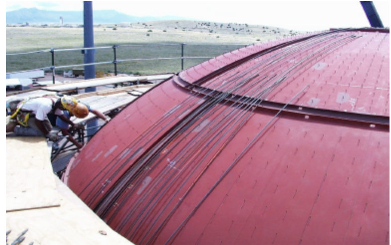
Figure 2.41 Installation of Inner Dome Rebar
