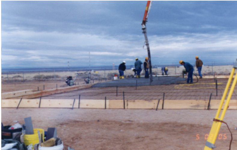
Figure 2.12 Placement of PCCV Mudmat
