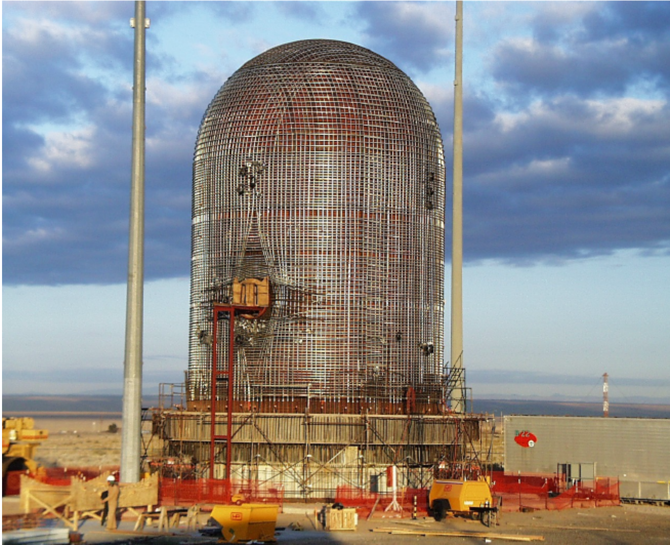
Figure 2.44 PCCV Model Tendon Sheaths
