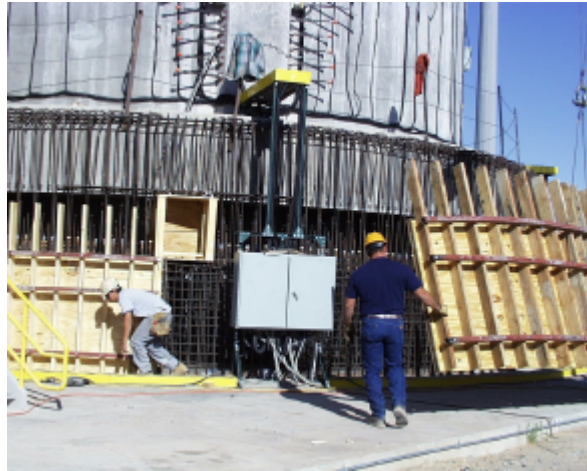
Figure 2.53 Final Basemat Concrete Lifts
