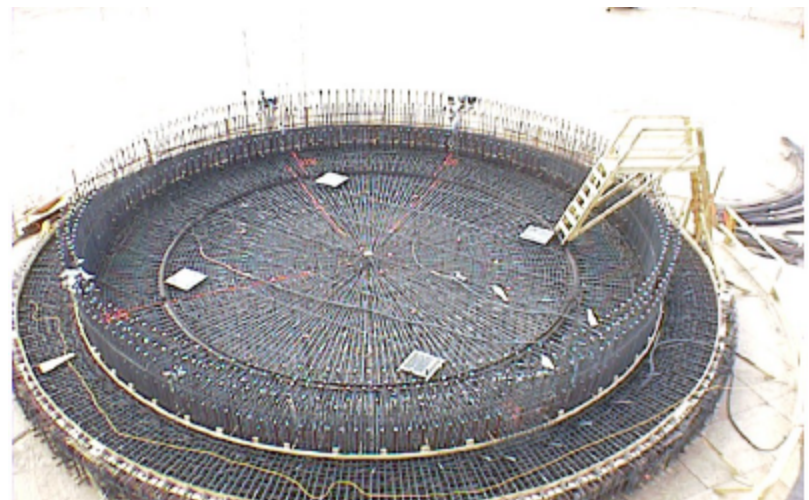
Figure 2.23 Basemat Top Rebar (F3) and Wall Dowels
