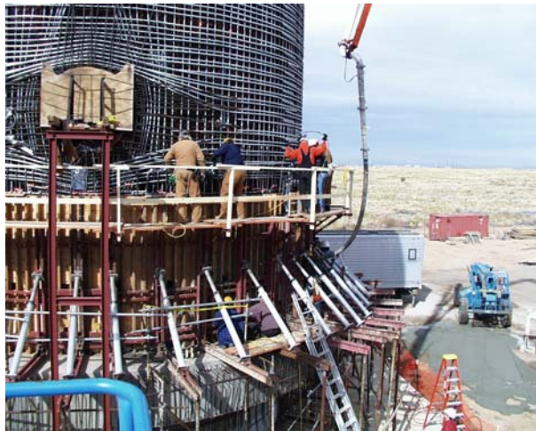
Figure 2.47 Placing C1 Concrete
