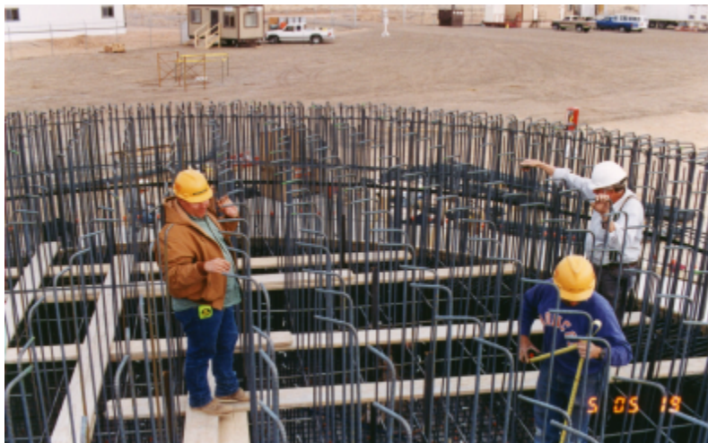
Figure 2.14 Basemat Bottom Bars and Vertical Ties
