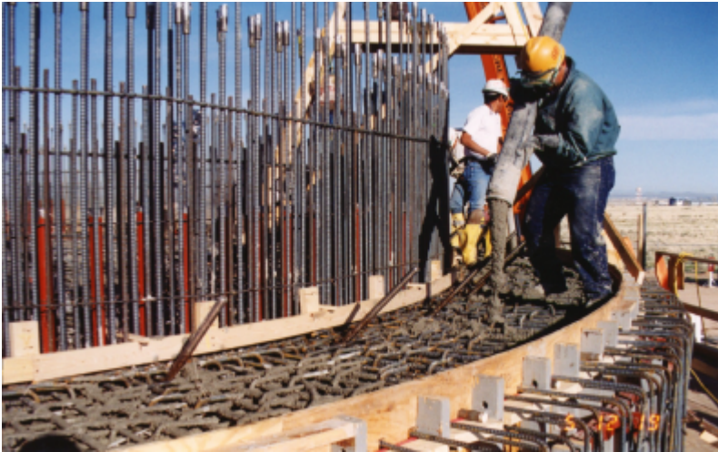
Figure 2.24 F3 Concrete Placement
