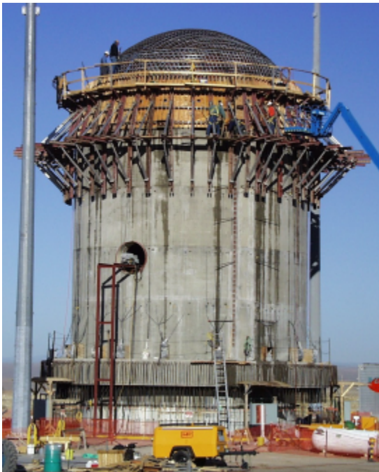
Figure 2.51 D1 Formwork Erection
