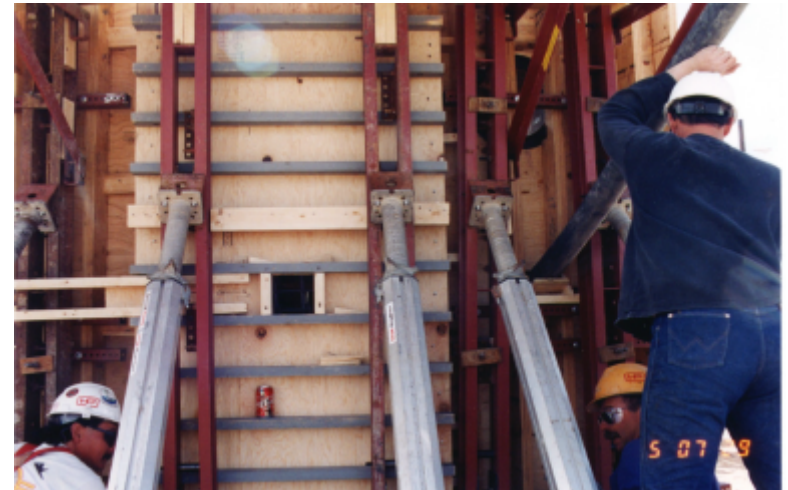
Figure 2.27 Wall Mock-up Form w/ Concrete 'Window'
