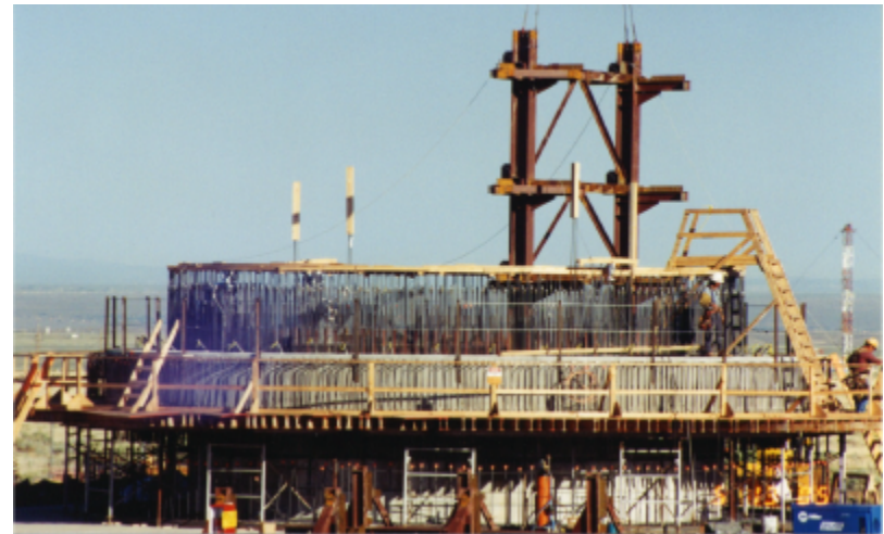
Figure 2.31 Instrumentation Frame Erection
