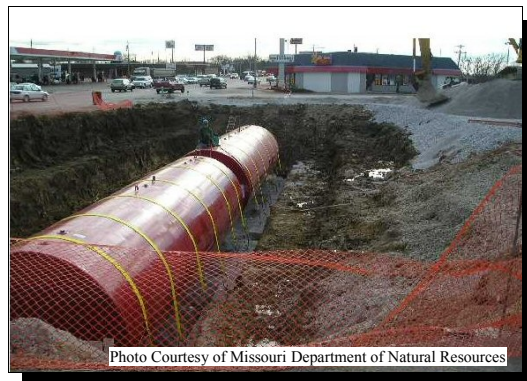
INSTALLATION OF AN UNDERGROUND STORAGE TANK
