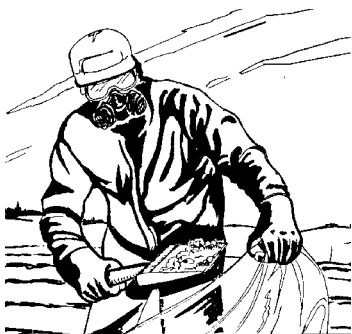
Figure 6-22. Shovel all the spilled material and absorbent into a leak-proof container or chemical resistant bag. Foam spills can be placed into the nearest manhole of the sewer line being treated.
