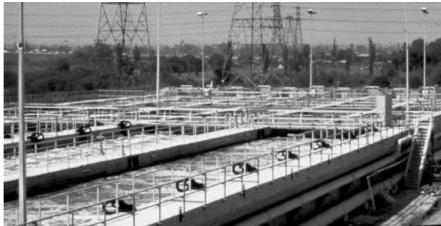
Figure 5-1. Sewer line root control pesticide applications can have serious impacts on wastewater treatment plants unless proper planning takes place before application.
