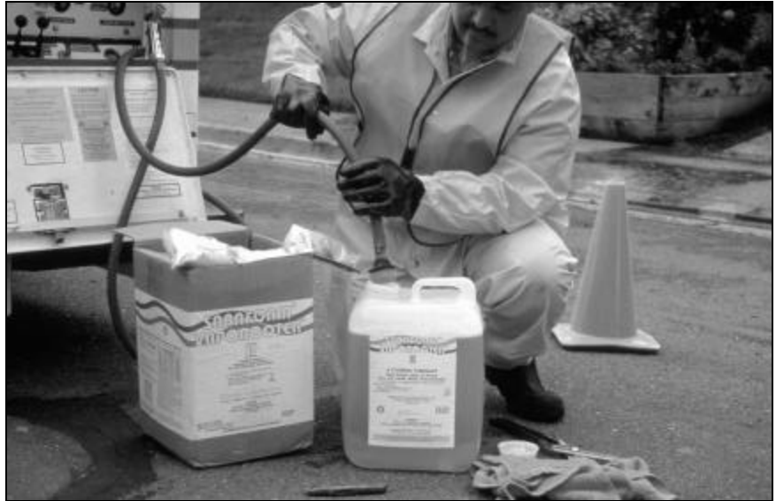
Figure 6-4. Proper personal protective equipment is needed to protect yourself from exposure to root control pesticides. This handler is wearing protective bodywear, waterproof gloves and boots, and a faceshield.
