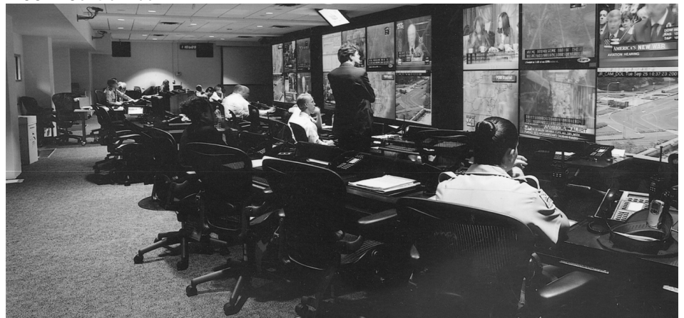
A CCTV Control Room
