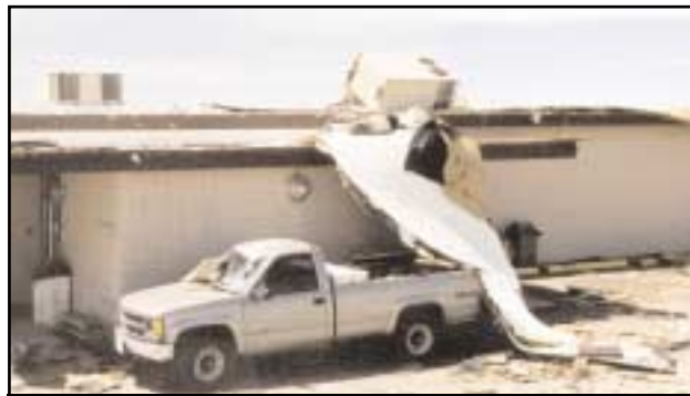
Portions of the Mercury's gas station and fleet operation's roof are blown off due to the high winds at the Nevada Test Site.
