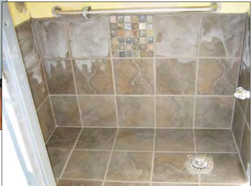
After: An almost-renovated bathroom will be much more sanitary and easy to maintain.
