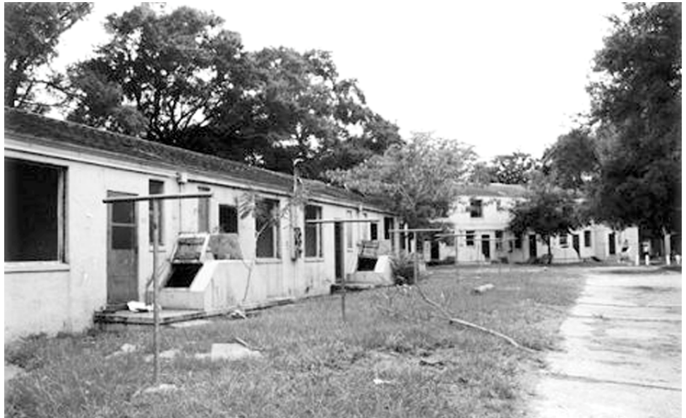
Before HOPE VI renovation
