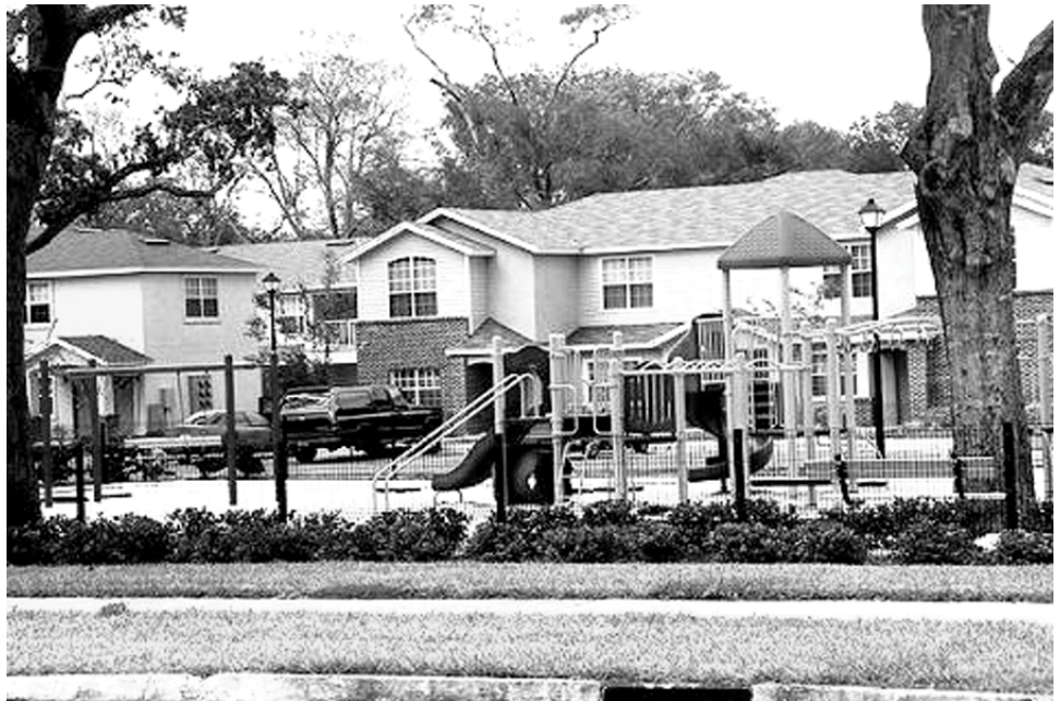
After HOPE VI renovation
