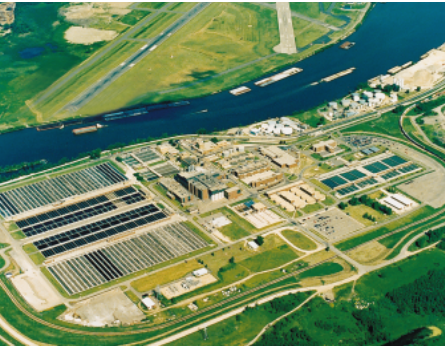
Figure 7-2. The Twin Cities (Minneapolis-St. Paul, Minnesota) Metropolitan Waste Treatment Plant was instrumental in improving water quality downstream to Lake Pepin. Prior to completion of secondary treatment capabilities in 1978, low dissolved oxygen led to declines in macroinvertebrate and fish populations. More recently, sanitary and storm sewers were separated to reduce waste discharge during heavy rains (Source: Kent Johnson, Metropolitan Council, Environmental Services).
