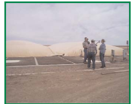
Anaerobic digester at a 5000-head swine farm in Colorado.
