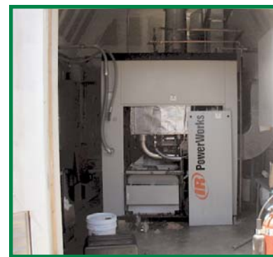
Entrance of the shed housing the IR PowerWorks™.
