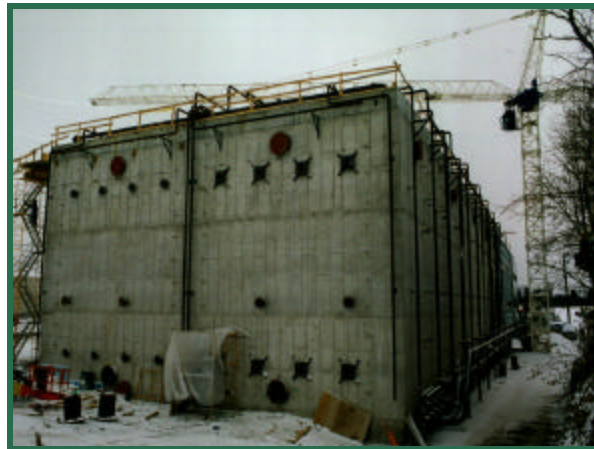
SUBBOR Waste Processing Digester Under Construction at Guelph, Ontario
