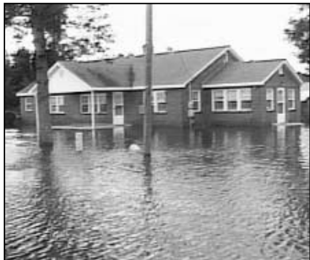
North Carolina flood caused by Hurricane Floyd, September 1999.
