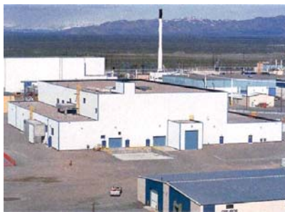
Fuel Processing Facility at the Idaho National Laboratory
