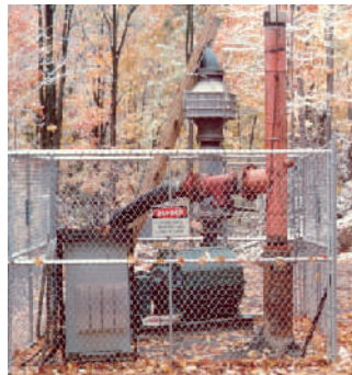
Gob Well, Pennsylvania. Photo courtesy of REI.
