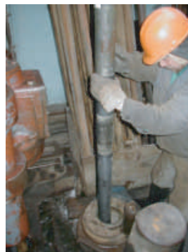
Lowering the Downhole Testing String.
