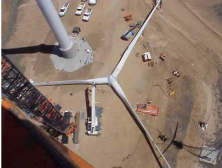
Figure 31. POC Turbine Rotor Being Installed
