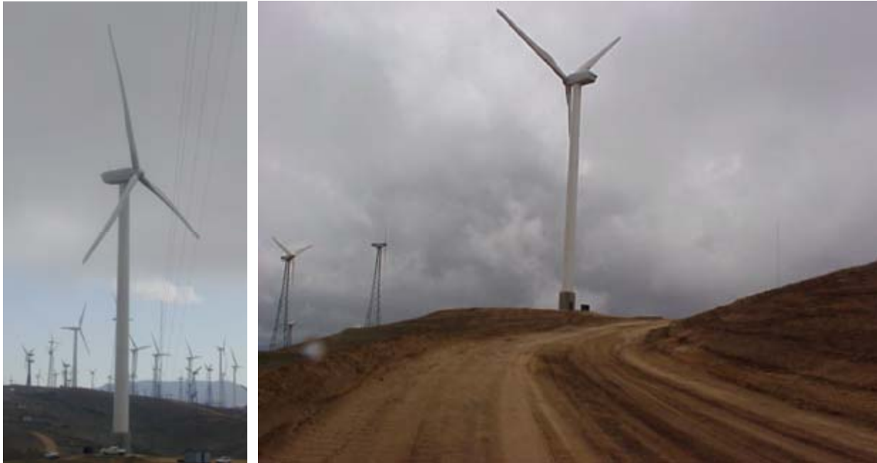
Figure 41. EMD Turbine Installed in Tehachapi, California
