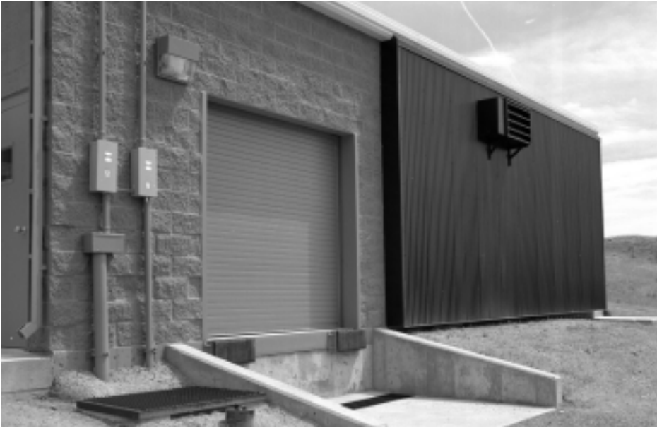
Figure 7. The transpired collector on the Waste Handling Facility at the National Renewable Energy Laboratory in Golden, Colorado.
