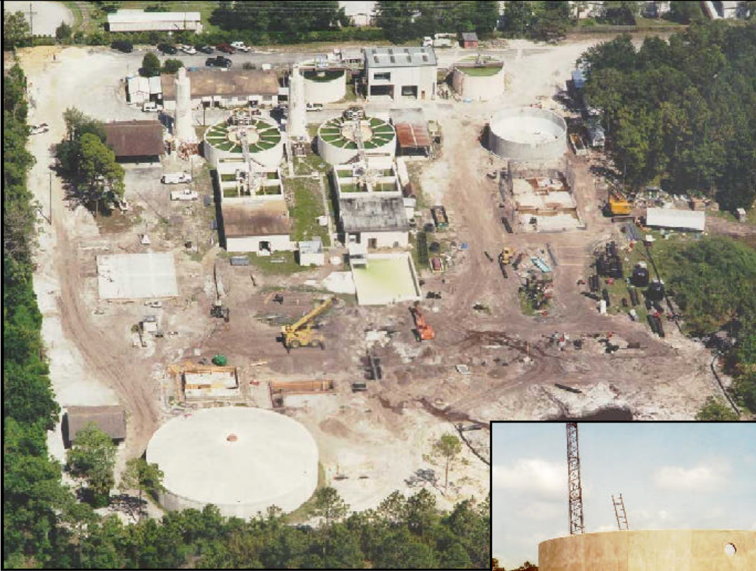
The City of Port Orange, Florida, received $9.1 million in DWSRF assistance to upgrade and expand its ground water treatment facility. Shown is an aerial view of the project site (left) and the construction of a new lime softening tank (insert).
