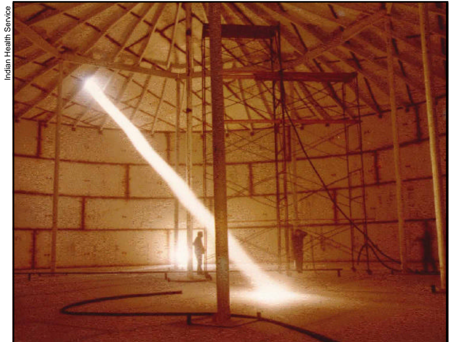
The construction of a treated water storage tank nears completion in Nuiqsut, one of the most northerly communities in Alaska. In many Alaska Native communities, water tanks and treatment plants must be elevated on pilings to prevent the heated facilities from subsiding into the permafrost.
