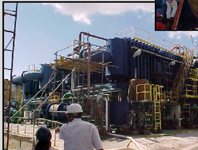
A water distillation plant, operated by the Virgin Islands Water and Power Authority, is shut down and disassembled for repair. Seawater is pumped through screens, then distilled to remove the salts and make the water potable. This facility also uses an ion separation process to extract chlorine from the seawater for use as a disinfectant.
