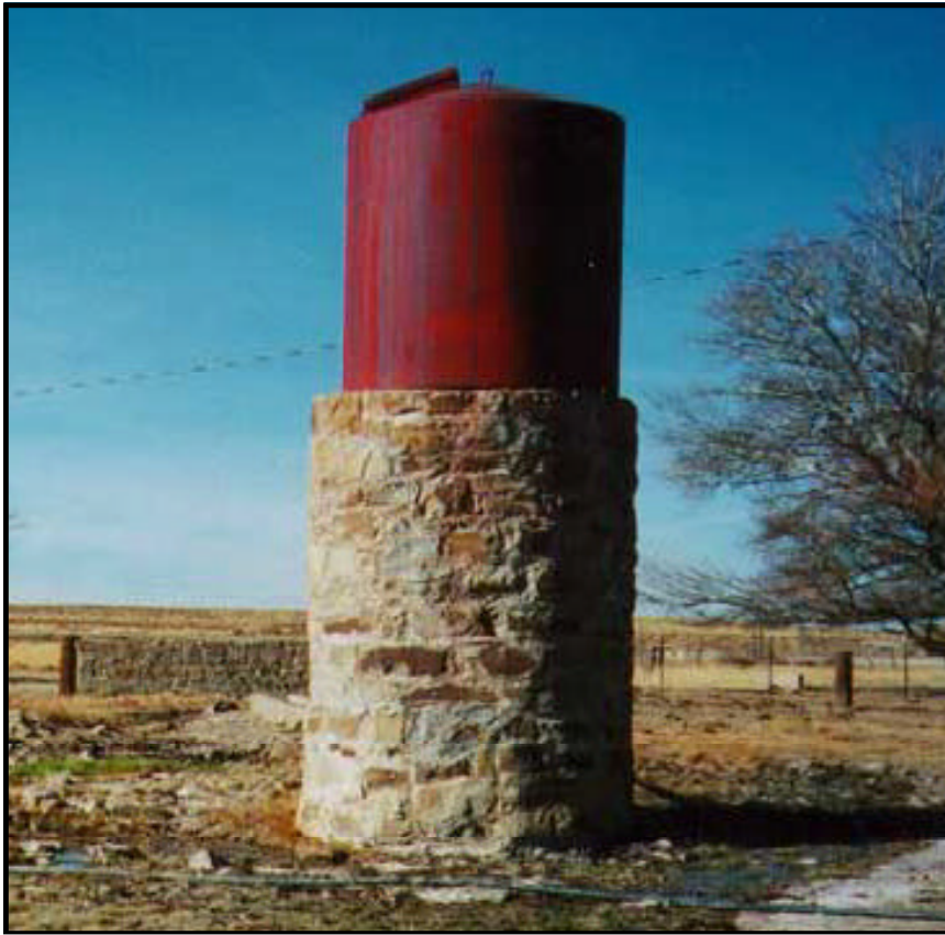
This 1,000-gallon storage tank is mounted on top of a stone structure to provide a pressure gradient.
