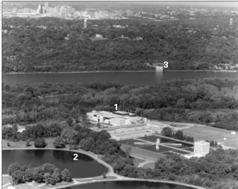
Cincinnati's surface water treatment plant was upgraded in 1995 to include deep bed carbon filtration. This process removes organic contaminants found in Cincinnati's source, the Ohio River. The treatment plant (1) and untreated water storage (2) are shown in the foreground. The intake (3) is shown on the opposite bank of the river. The city and elevated finished-water storage tanks can be seen in the background.
