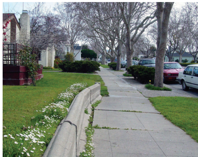
Figure 2-4. View looking east along an offset wall and sidewalk on 6th Street in Hollister adjacent to Dunne Park. The park itself preserves a low hill that is a scarp of the Calaveras Fault. The low area within the park west of the scarp was in part a sag pond prior to development of the area.
