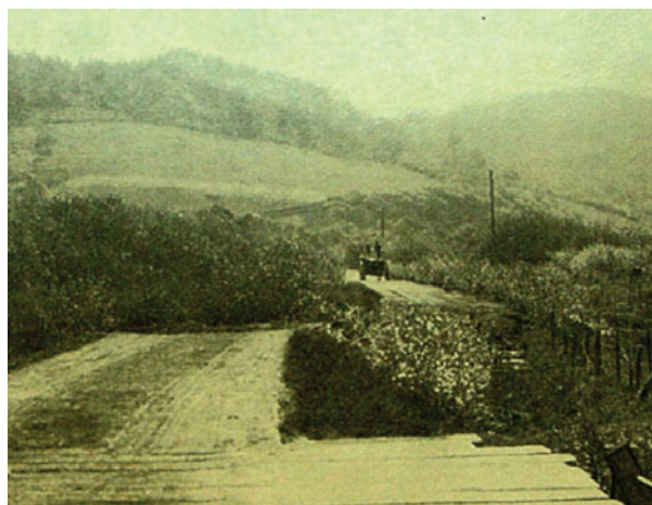
Figure 9-6. This view of an offset road near Point Reyes Station shows 20 feet (6 m) of horizontal slip caused by the 1906 earthquake. Photograph by Gilbert (1908).
