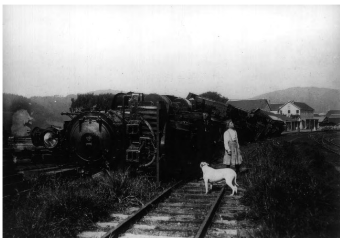
Figure 9-3. A famous historical photograph taken by an engineer of a derailed train that tipped over at the Point Reyes Station during the 1906 earthquake (image from Jordan, 1907). The narrow gauge train was stopped at the station on a section of track that ran roughly parallel to the fault less than a mile east of the rupture. Based on the engineer's description of the rocking motion that fell the locomotive, Anoshehpour and others (1999) calculated the earthquake motion created ground acceleration that was in the range of 0.7 to 1.1 g ( g is the force of gravity).
