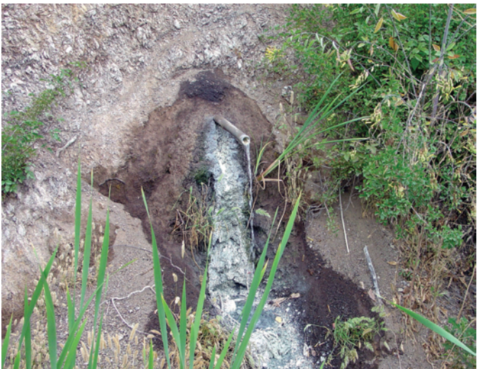
Figure 2-18. A drain pipe in the Santa Cruz Mudstone near the fault zone is a source of sulfur-rich water. Sulfur and mineral springs are common along faults throughout the region. Warning! Do not attempt to have field trip participants cross the road to examine the springs or outcrops. There isn't enough room to stand next to the road. Rather, a single individual might carefully cross the road and fill a water jug. However, the rotten-egg smelling water is not safe to drink. Cattails grow in abundance near the springs.
