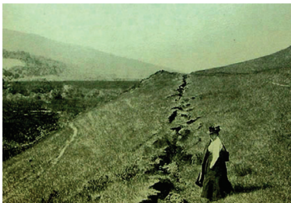
Figure 9-4. Photograph by Gilbert (1908) of surface rupture along the fault near Point Reyes Station. The view is looking northwest toward marshlands at the south end of Tomales Bay. The photograph illustrates a classic example of a sidehill bench. Note the extent of timber removal on Inverness Ridge in the distance (top left).
