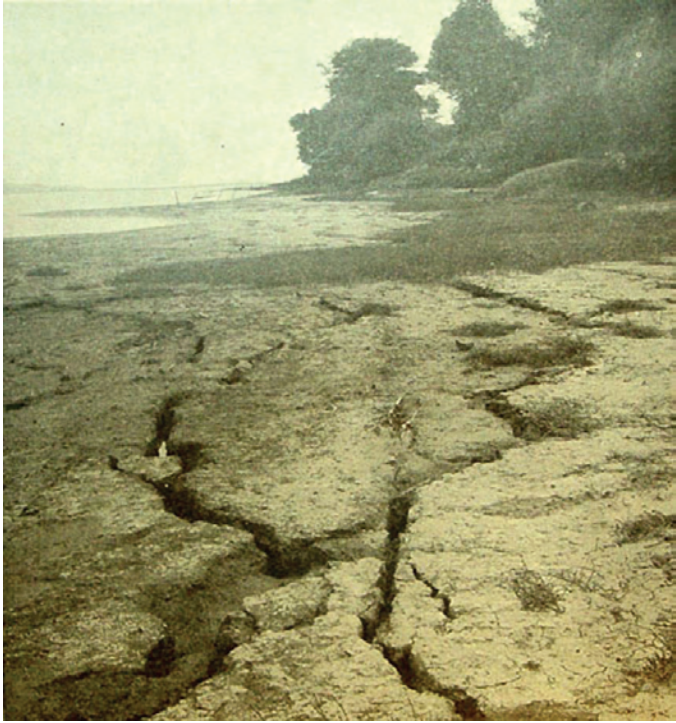
Figure 9-44. These cracks along the shore of Bolinas Lagoon formed during the 1906 earthquake. Photograph by G. K. Gilbert (1908). This view is looking southeast along the western shore of the lagoon toward what was then the undeveloped barrier spit that is now home to Stinson Beach.
