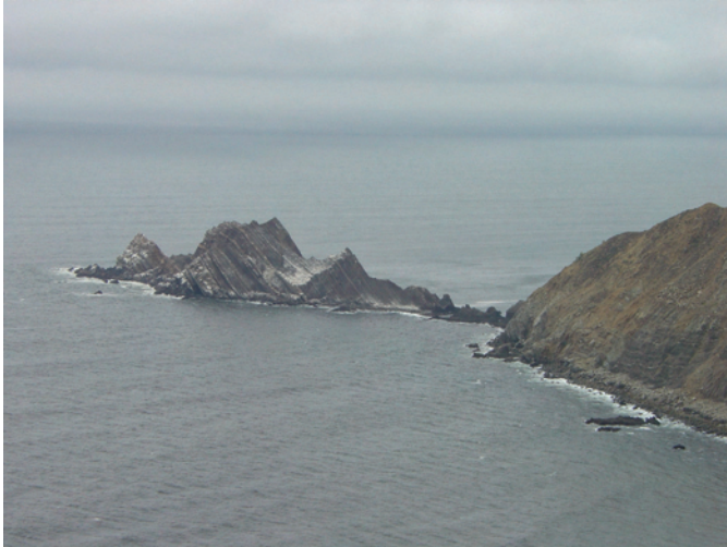
Figure 8-17. Pedro Rock at the south end of Point San Pedro consists of steeply dipping beds of Paleocene-age sandstone and shale (covered locally with bird guano). Darrow (1963) described unconformable relations between the Paleocene sedimentary rocks and sedimentary rocks of late Upper Cretaceous beds on San Pedro Point (to the right). Whether these Upper Cretaceous sediments are in conformable contact with the Salinian granite is unclear. A remnant of the old Ocean Shore Railroad bed is visible along the shore (lower right).
