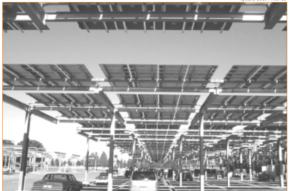
This solar electric system in Sacramento, California, generates enough electricity to meet the needs of about 180 homes. While providing electricity, it also shades part of the Cal Expo parking lot. The largest parking-lot solar system in the world, this project was a joint effort of the Sacramento Municipal Utility District and DOE through the TEAM-UP program.
