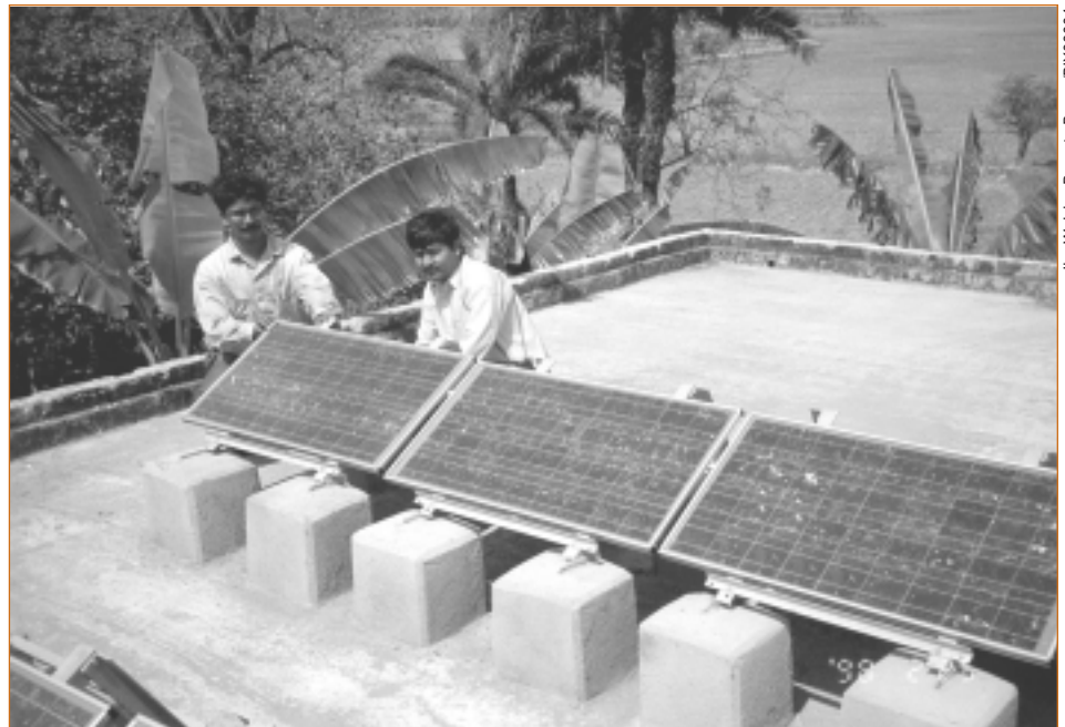
Local technicians install solar electric modules on a village clinic as part of a collaboration between the NCPV and the Solar Energy Center in New Delhi, India, to test U.S. thin-film solar modules.
