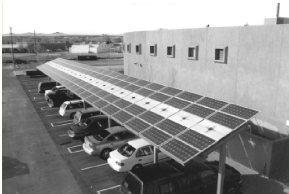
This solar electric system installed in FY 1999 delivered about 23 megawatt-hours of electricity to the Indian Pueblo Cultural Center in Albuquerque, New Mexico, in its first year of operation. NCPV engineers at Sandia conducted the project's electrical design review and monitor system performance.
