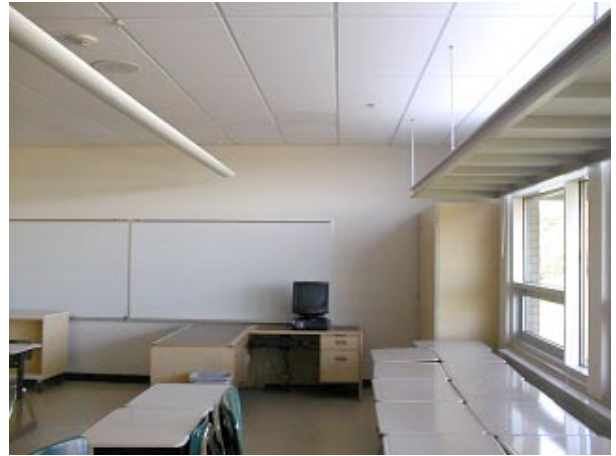
Classroom view shows how the outside light “bounces” into the room off the light shelves inside the room.
