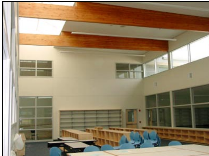
The clerestory and spun fiberglass skylight provide ample light in the media center.
