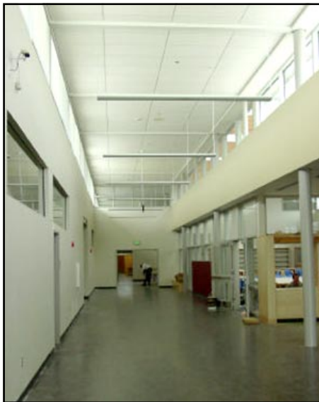
Clerestories in the 18-foot high hallway provide natural daylighting with uniform light levels within the hall.
