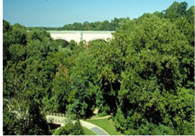
View of the Calvert Bridge, spanning across Rock Creek Park Photograph courtesy of the DC SHPO
