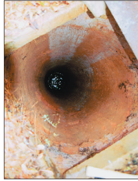
In parts of Rockdale County, ground water is obtained from large-diameter bored or dug wells. Ground water seeps into the well and collects at the bottom where it can be withdrawn (above, right). A bored or dug well is more susceptible to drought conditions than a deep drilled well. The sides of the bored well, shown in the photo above, are formed from saprolite derived from weathering of granite gneiss. Photo by Lester J. Williams, USGS.
