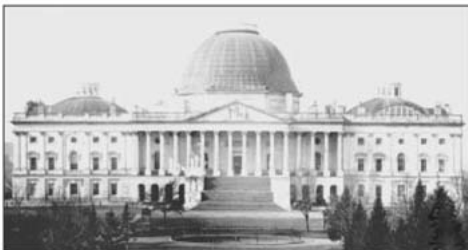
The Capitol in 1846. The building before addition of the new wings and dome. Library of Congress
