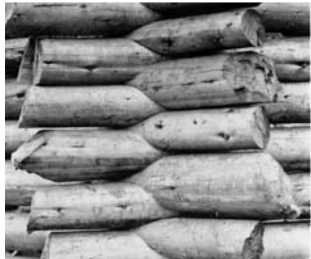
The log work on the corners of the Lake Ranger Station. 1923.
