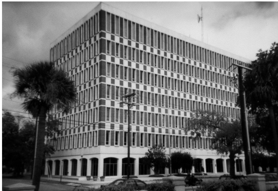
Figure 3: Example of Vacant GSA-Owned Property—the L. Mendel Rivers Federal Building in Charleston, South Carolina
