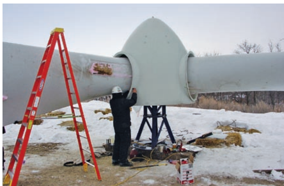
A technician prepares the Vestas V-47 turbine for installation.
