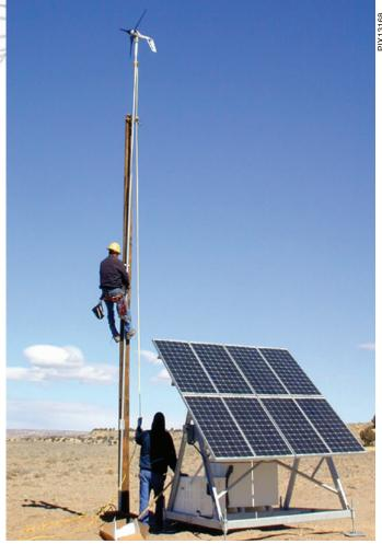
NTUA's technicians plan to install 63 hybrid systems this year to provide power for remote Navajo homesteads.
