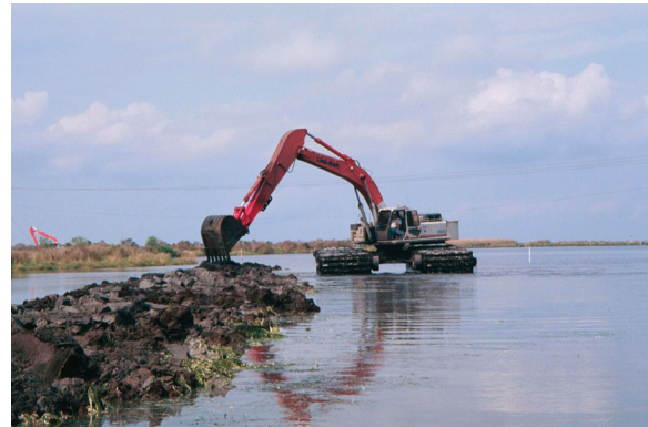
Terrace construction. — Ducks Unlimited
