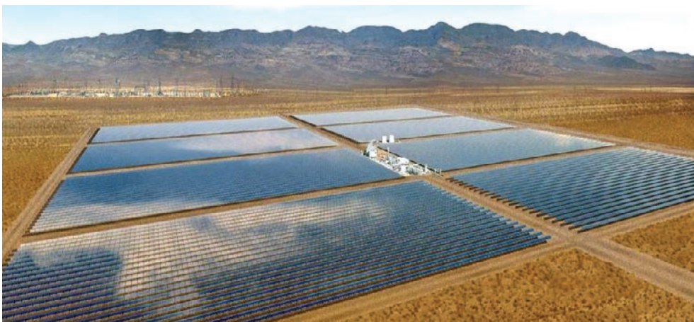
64-megawatt solar plant in Boulder City, Nevada.
