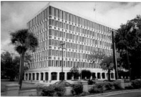
Figure 25: Federal Office Building, Charleston, South Carolina
