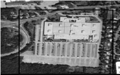
Figure 24: IRS Service Center, Andover, Massachusetts
