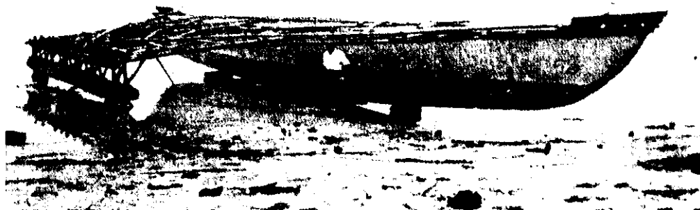
Fig. 5.4. Gilbertese 100-foot baurua under construction at Tabiteuea in 1939. (Photo by H.E. Maude)
