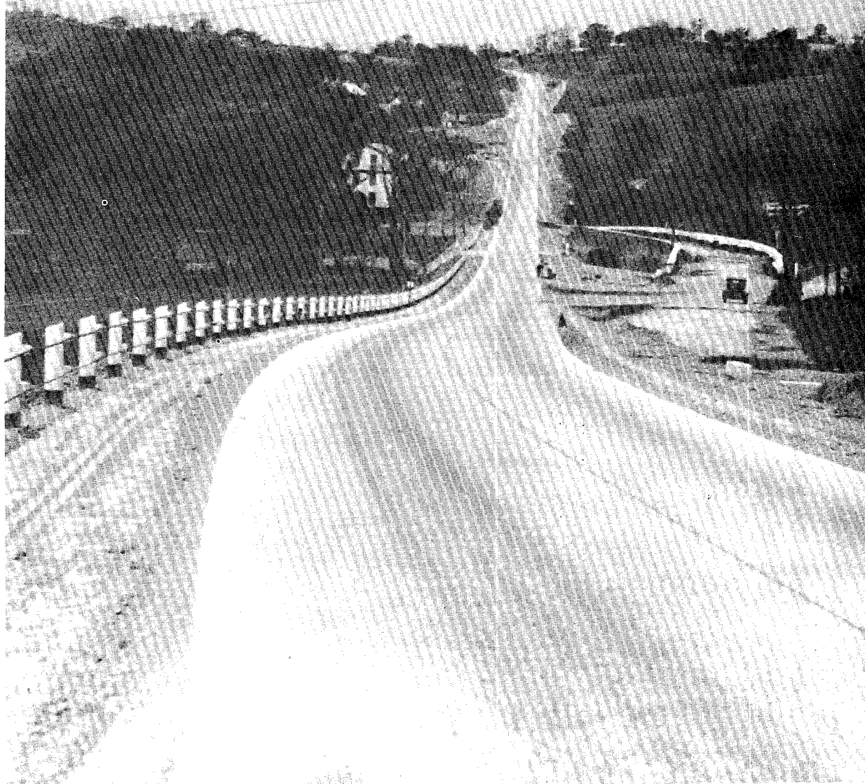
National Road: S-Bridge, 1818, U. S. Route 40, Six miles west of Washington, Pennsylvania. The bridge appears today as shown in this 1931 photograph.
