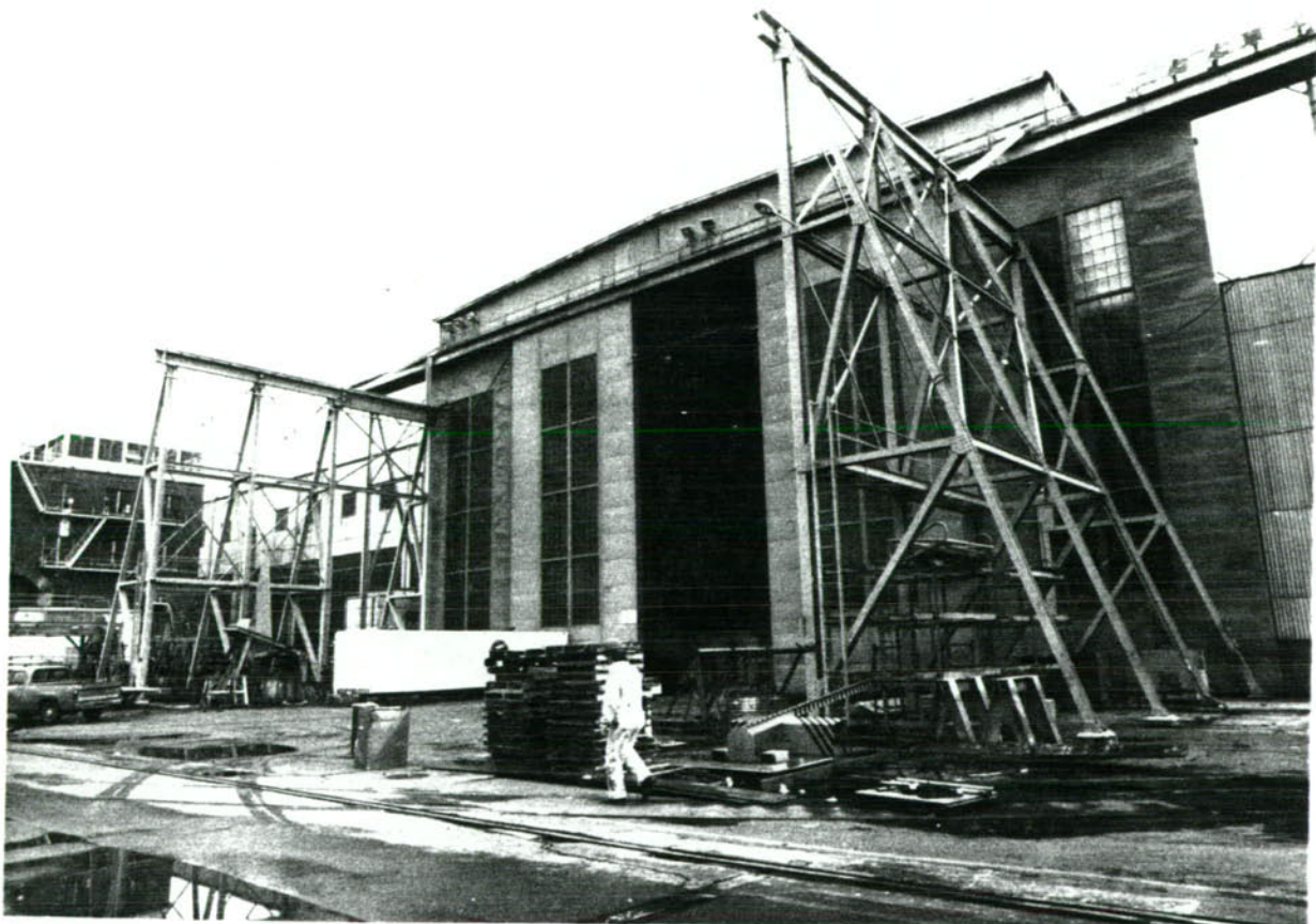
8. Another view of the large, L-shaped shopfitters building.
