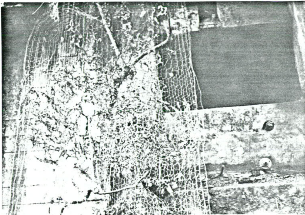
7. Second-floor opening of a large, igloo-type magazine on Makhnati Island. Note the chicken wire and fragments of burlap that camouflaged the face of the magazine.
