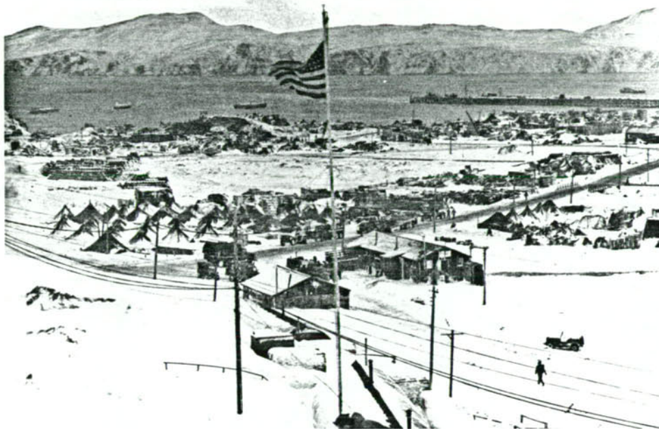
9. An American Camp on Kiska. Note the new dock constructed by U.S. Army Engineers. December 9, 1943.
