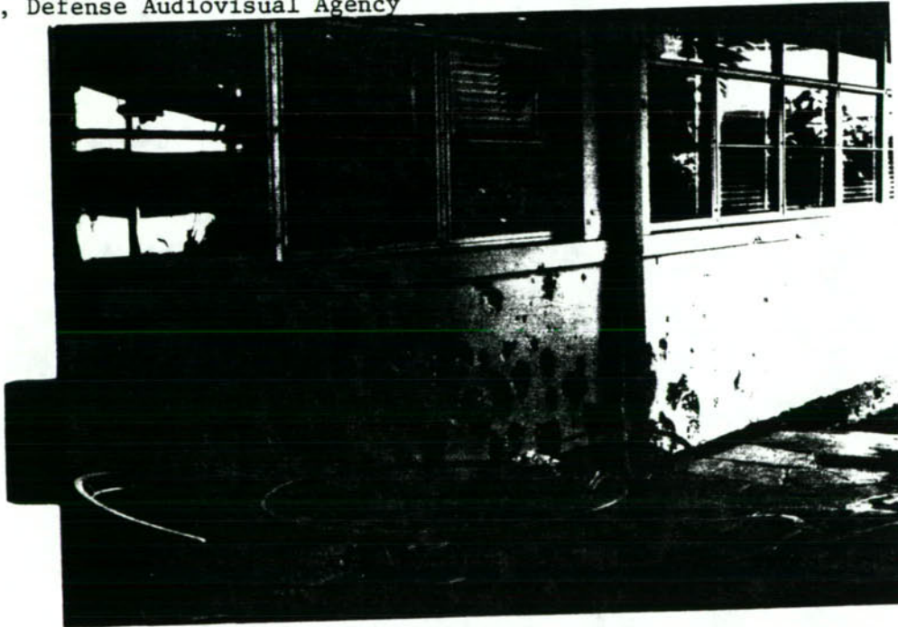
6. Bullet holes still pockmark the barracks' walls. The structure now is an administrative building.
