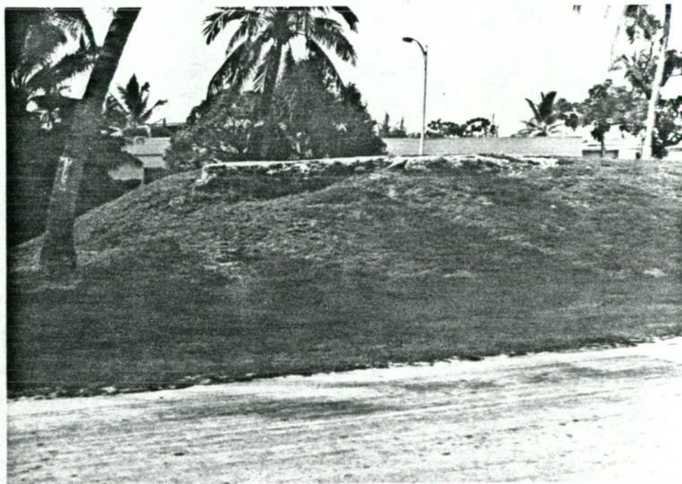
10. Japanese twin-mount, dual-purpose 127mm gun emplacement at the north end of Kwajalein Island, one of the last positions to be captured. Because of the island's low elevation, the Japanese constructed mounds for these weapons. This is called "Bunker Hill."
