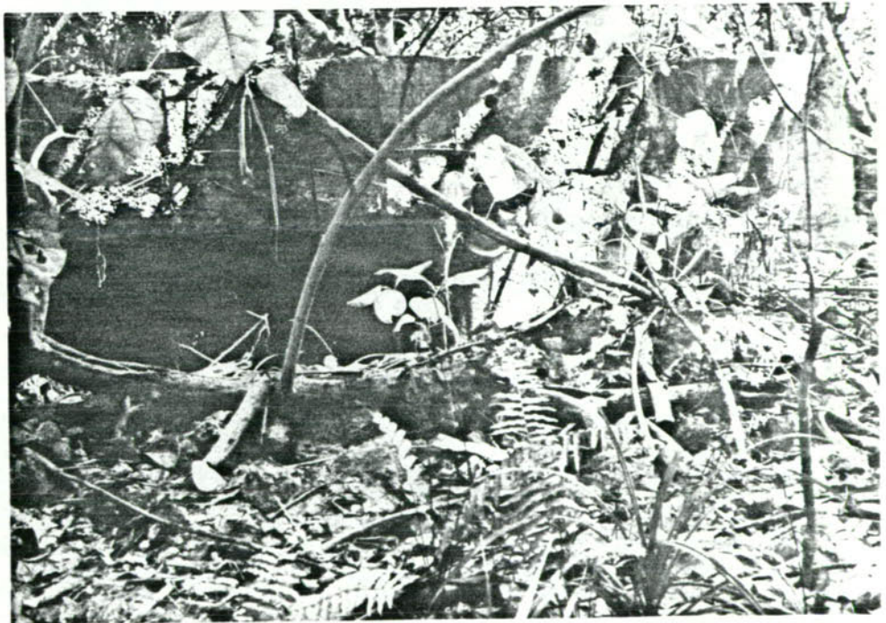
5. One of many coral and concrete pillboxes hidden in the jungle along the landing beaches. This one is inland from Beach White 2.
