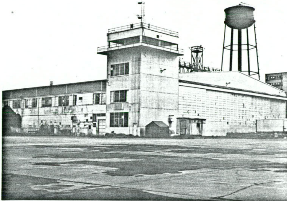
1. Sitka Naval Air Station. One of two hangars and control tower. The paved area in front was both aircraft parking and a short runway fitted out like an aircraft carrier's flight deck.
