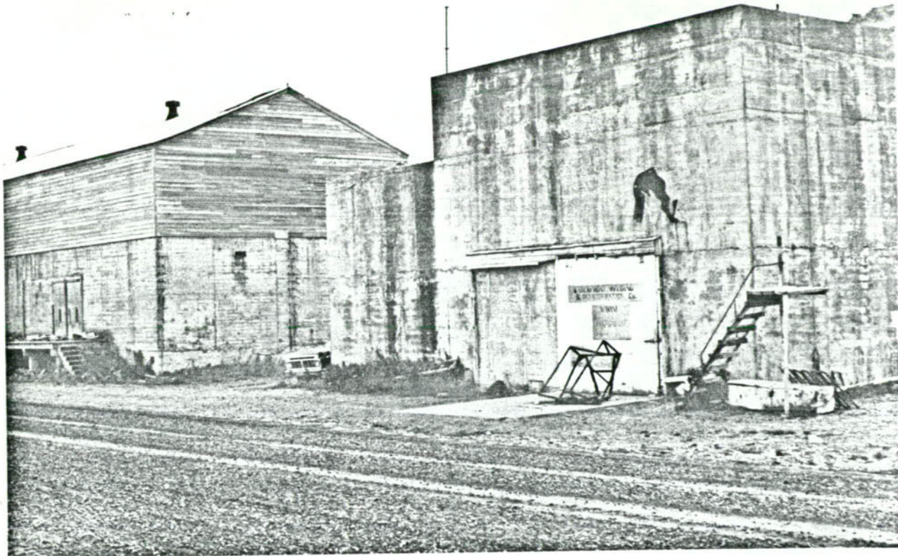
10. Torpedo assembly building on left; annex shop on right. Nearby are two torpedo explosives tunnels cut into hillside, Dutch Harbor.
