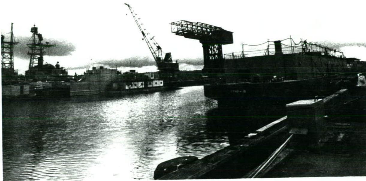
1. Pier 6 on left. The huge, revolving hammerhead crane to the right can lift the guns and gun turrets of battleships.
