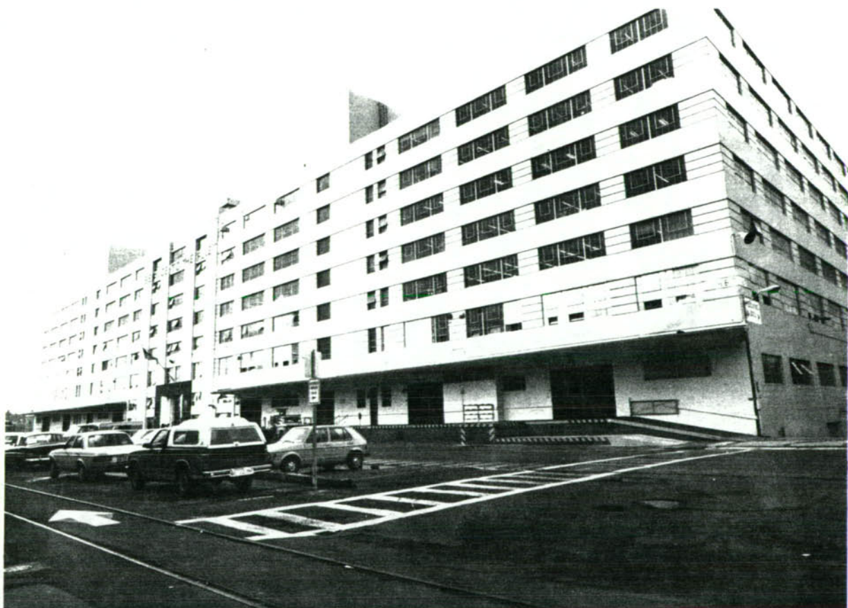
4. Huge supply building constructed at the shipyard during World War II.
