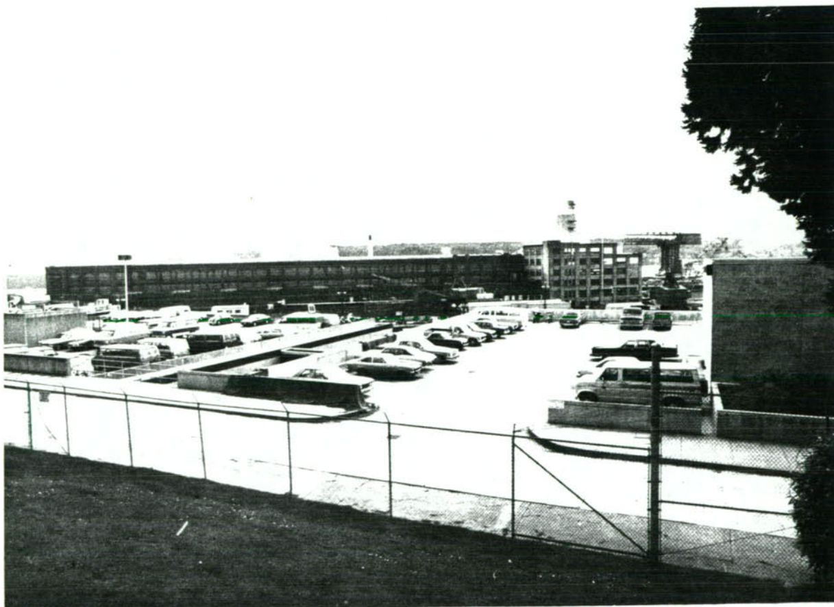
2. Machine shop building. The six-story extension on the right was added during World War II.
