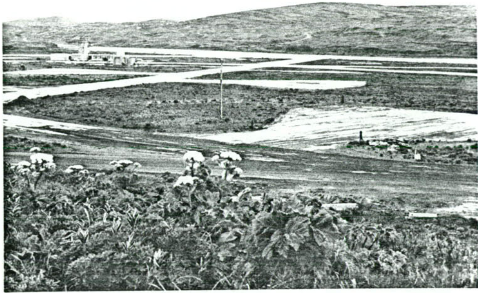
7. The army airfield constructed on Adak in September, 1942, for the Aleutian campaign has been much improved and is still used by naval patrol planes at Adak Naval Station. In the foreground are three of four hardstands that probably mark the sites of four Kodiak T-type hangars of World War II.
