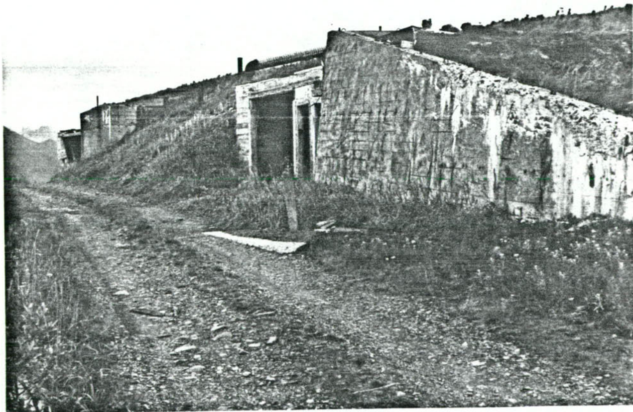
6. Casemated, reinforced-concrete magazines for 8-inch coastal gun battery high on Ulakta Head.
