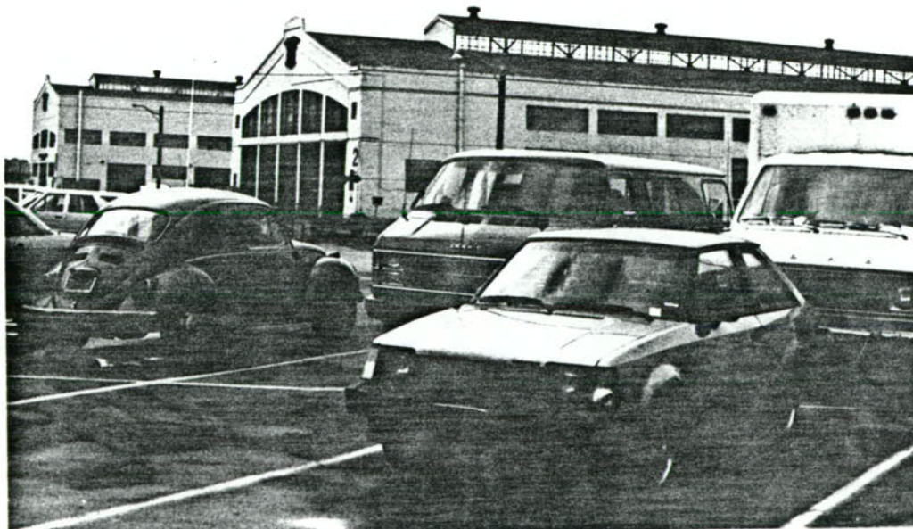
4. Piers 1, on left, and 2, San Francisco Ports of Embarkation. The shed on Pier 2 is the original, permanent shed. Pier 1's shed was reconstructed in the 1930s.
