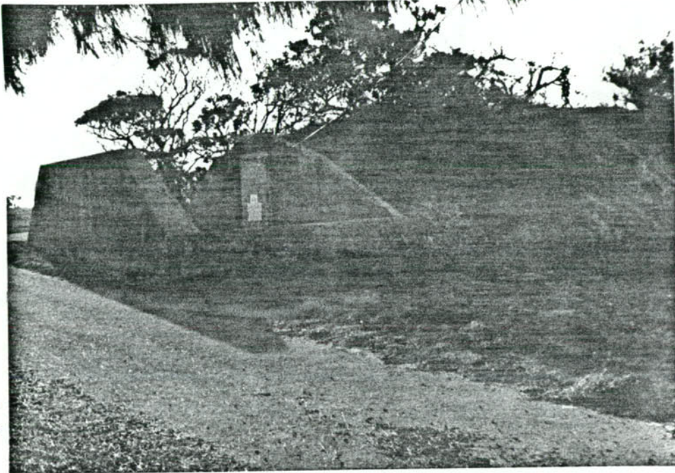
2. Entrance to an American igloo-type magazine. In December 1941, two of these magazines served as hospitals, one was the Marines' command post, and only the fourth continued to store aerial bombs. Only three remain.
