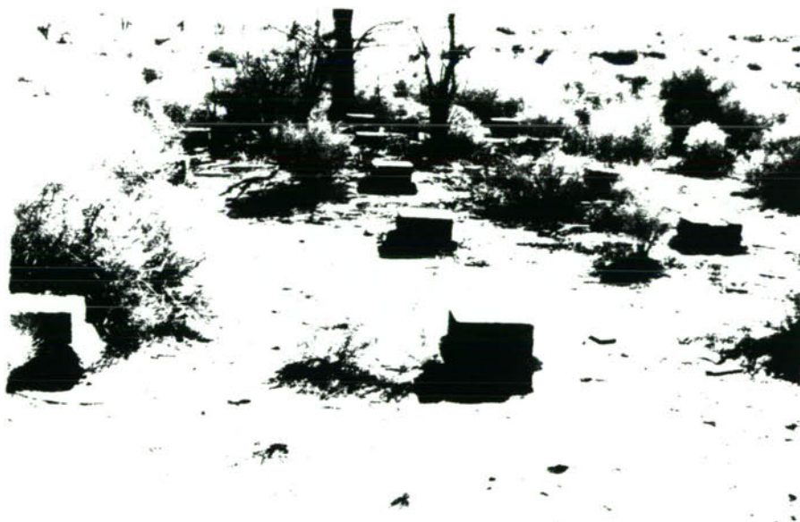
9. Concrete foundation posts slowly weather away in the desert at Manzanar.
