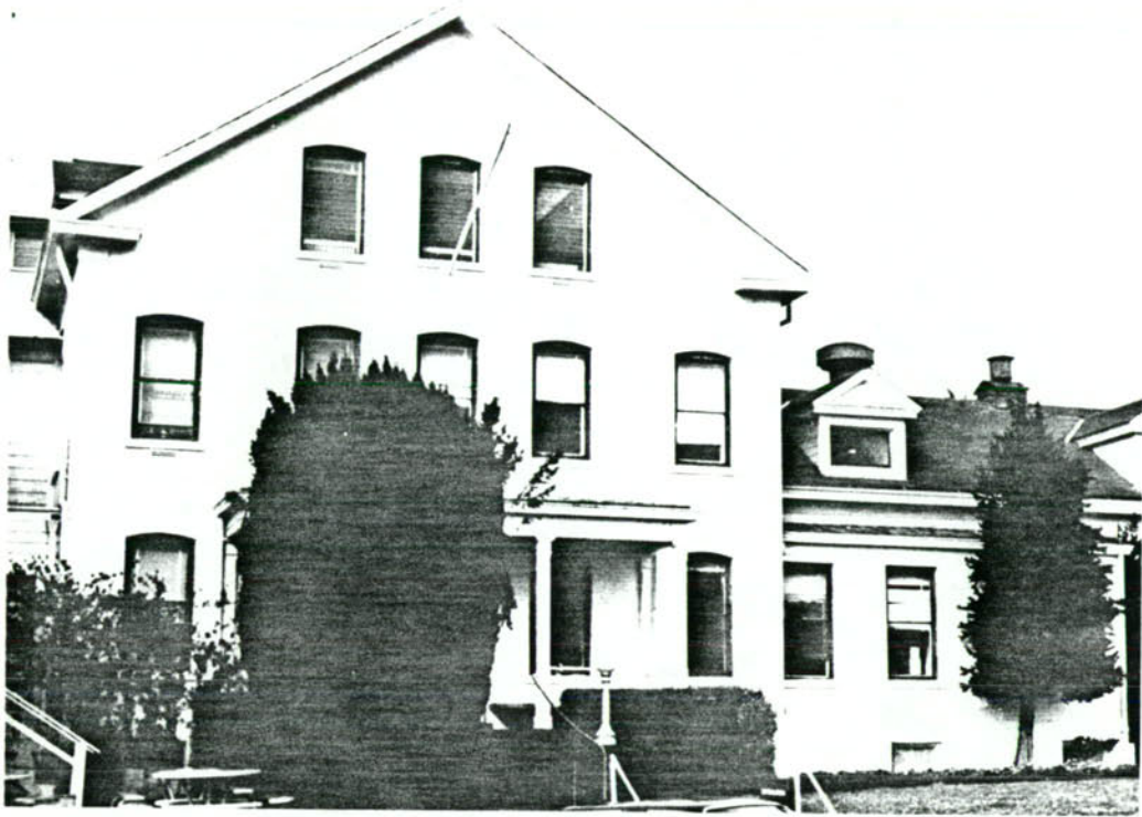
1. Brick portion of the headquarters building, San Francisco Port of Embarkation, Fort Mason. The U.S. Army constructed this unit as a posh hospital in 1902.
