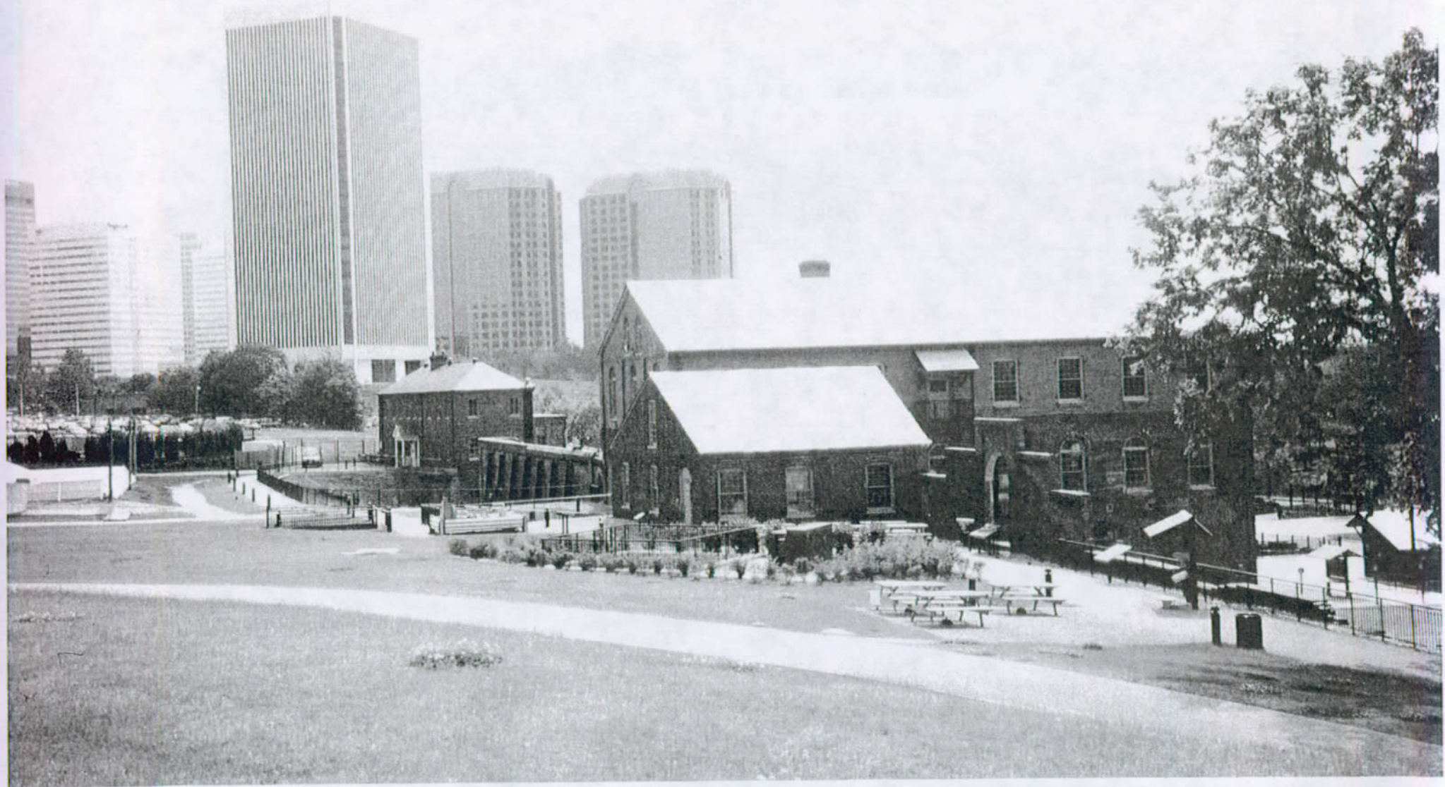
TREDEGAR IRON WORKS - DOWNTOWN RICHMOND
