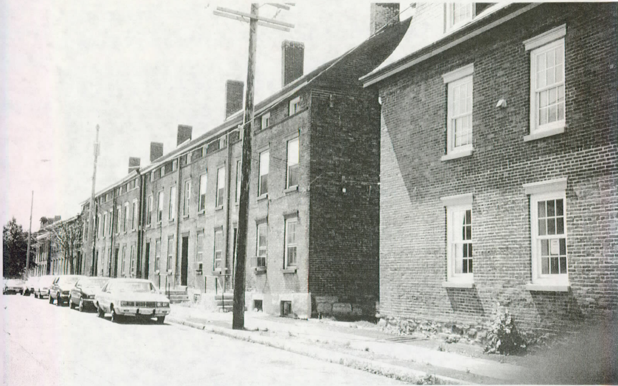
HARMONY MILLS - WORKERS' HOUSING
