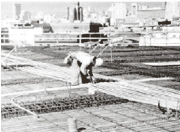
Figure 2-1.3. Worker installing pipe on deck
