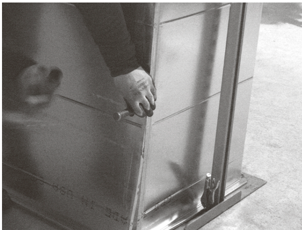
Figure 2-5.2. Tacking duct together
