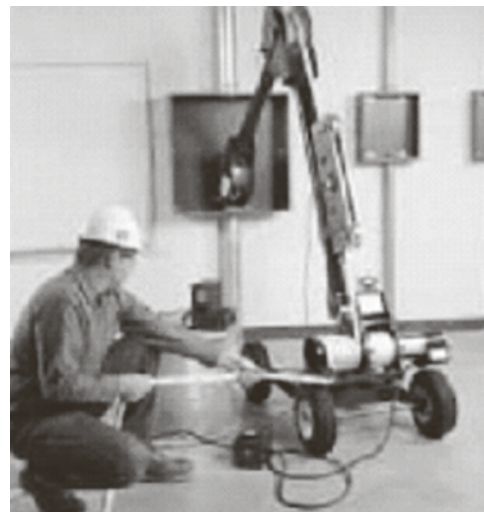
Figure 2-1.4. Worker operating cable tugger/puller
