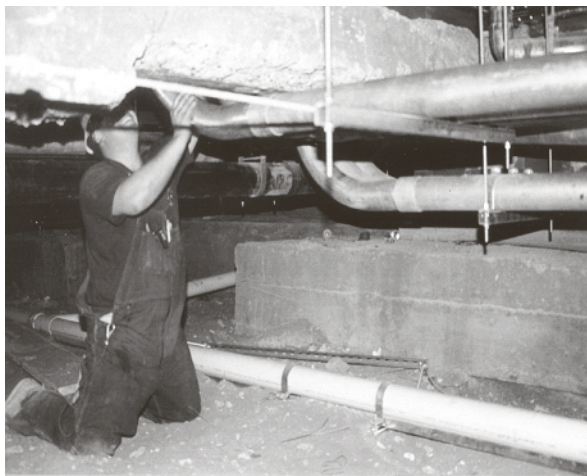
Figure 2-1.1. Worker installing pipe
